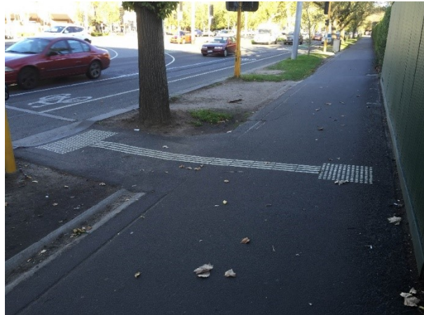
Figure 37: Example of guidance strip used to guide pedestrians with vision disabilities to a midblock crosswalk in Melbourne, Australia.
