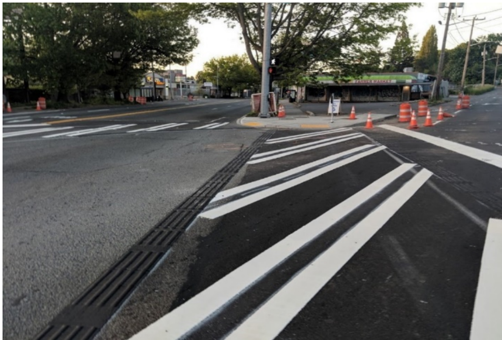
Figure 20: The City of Seattle used guidance strips to help people with vision disabilities maintain their orientation through this crosswalk at skewed intersections. This toolkit recommends crosswalk delineator strips (rather than guidance strips) in this situation, since some people with vision disabilities interact with guidance strips by walking on top of them. This toolkit also recommends that crosswalk delineator strips be of a contrasting color to adjacent surfaces. (Source: Dongho Chang)
