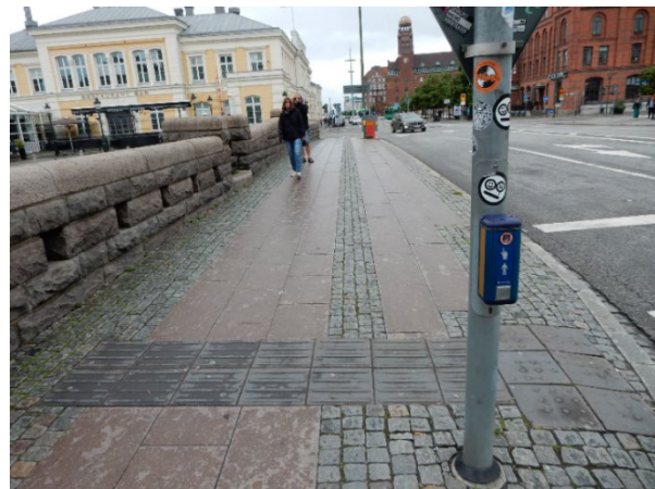
Figure 8: Example from Malmo, Sweden showing how detectable changes in surface texture and tactile walking surface indicators can be used to provide tactile guidance to people with vision disabilities. The pedestrian access route is defined by a smooth surface with rougher surfaces on either side. In addition, a detectable guidance surface is arranged perpendicular to the pedestrian access route to guide people with vision disabilities to the mid-block crossing. A detectable warning surface indicates the end of sidewalk space and the beginning of the crosswalk. (Source: Tony Hull)
