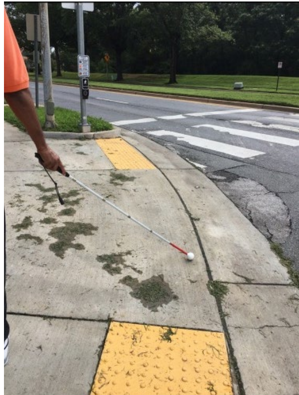
Figure 12: Example of a wrap-around depressed curb in Montgomery County. There are detectable warning surfaces at the crosswalk but not in other parts of the depressed curb.
