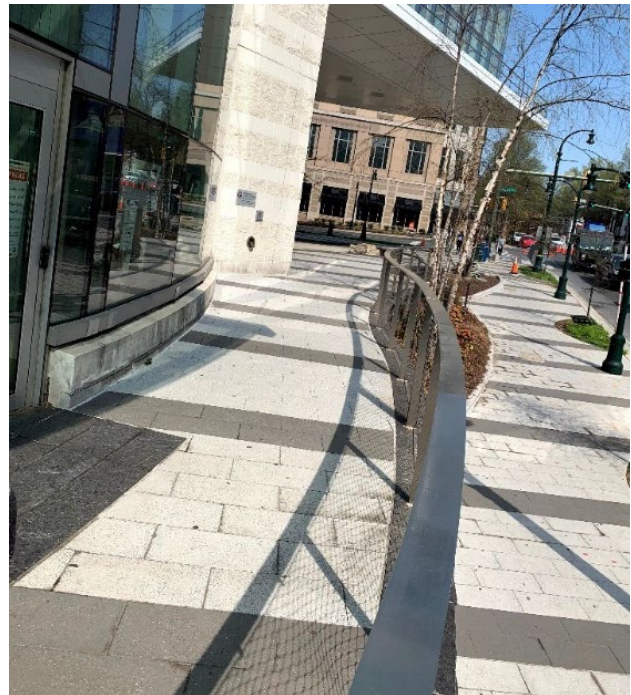
Figure 21: People with low vision sometimes misinterpret a pattern of parallel light and dark colored bars like this as steps. The bars in this photo, taken near the main entrance to the Silver Spring Public Library, are purely decorative and serve no navigational purpose.
