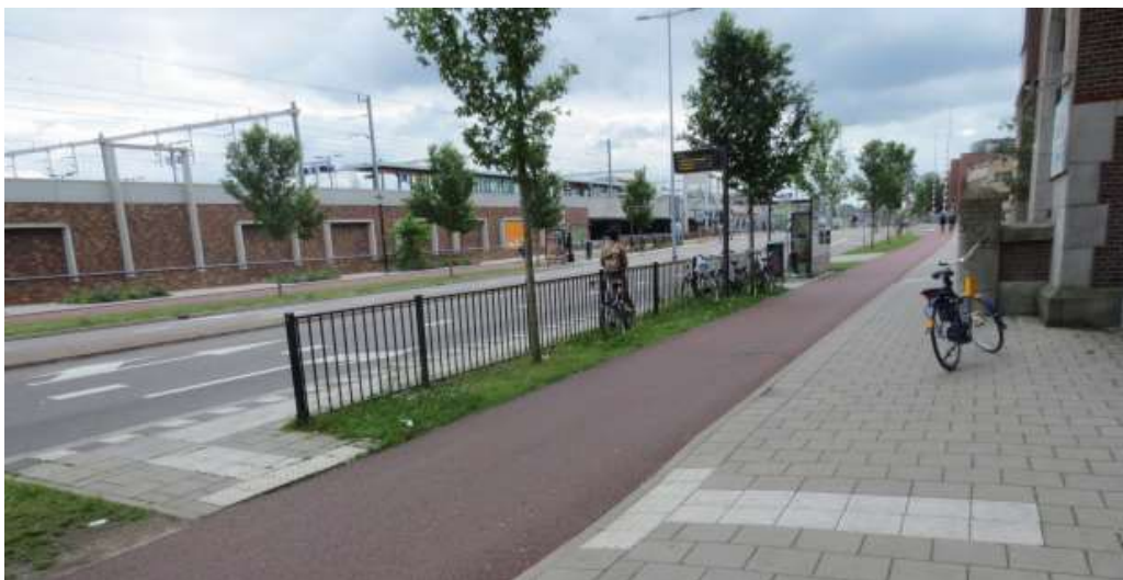
Figure 14: Example of guidance strips used to direct pedestrians with vision disabilities to a floating bus stop in the Netherlands.
