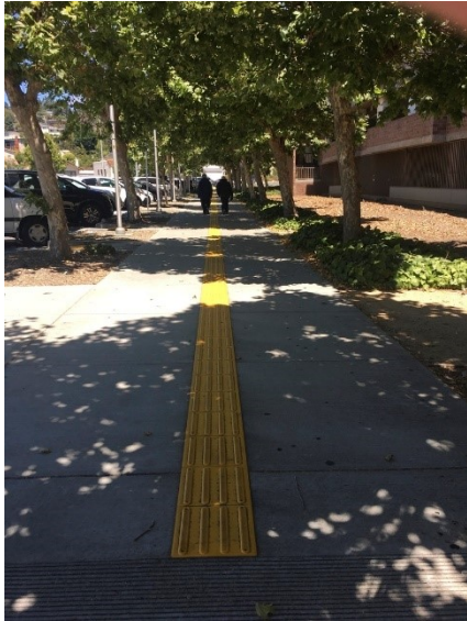
Figure 18: Guidance strips have been installed around the San Francisco Bay Area to help people with vision disabilities locate and navigate through BART transit stations. The images above are from a transit station in Contra Costa County. The indicators begin on the sidewalk about a block away from the station entrance and define a continuous path from the sidewalk, through the turnstiles, to the escalator and ultimately to the platform.
