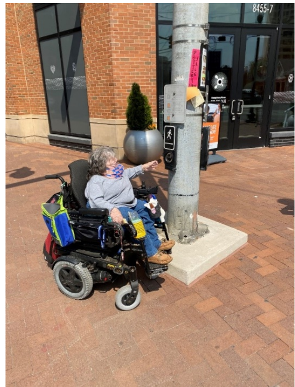
Figure 27: Person in wheelchair can't reach APS pushbutton button due to large concrete base.
