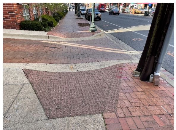
Figure 50: View of ramps to driveway between Safeway and 1810 Fenton Street.
