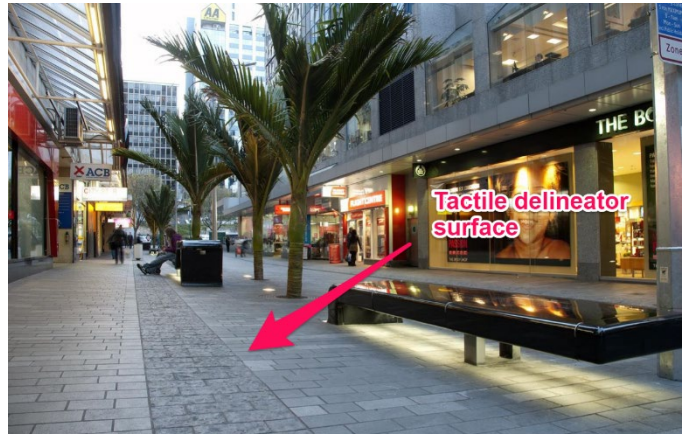
Figure 9: Example of a tactile delineator surface used in a shared space design in New Zealand (Source: Auckland Design Manual)
