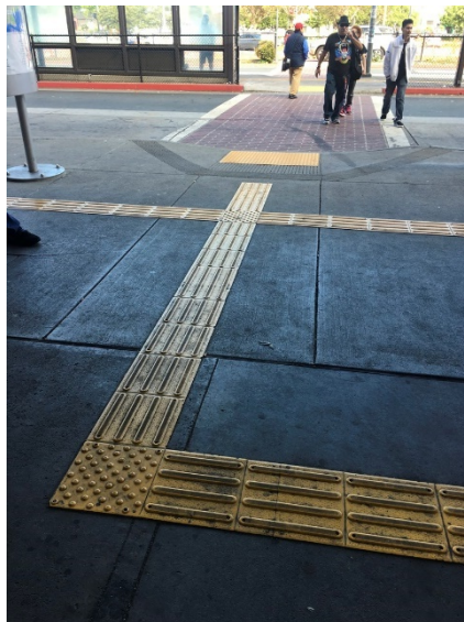
Figure 18: Guidance strips have been installed around the San Francisco Bay Area to help people with vision disabilities locate and navigate through BART transit stations. The images above are from a transit station in Contra Costa County. The indicators begin on the sidewalk about a block away from the station entrance and define a continuous path from the sidewalk, through the turnstiles, to the escalator and ultimately to the platform.
