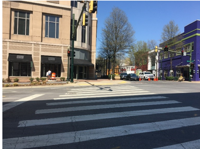
Figure 35: This crossing of Wayne Avenue at Fenton Street is both relatively long and skewed. In addition, there are wrap-depressed corners at both ends. These characteristics can make it difficult for a person with a vision disability to align properly to and maintain the correct heading when in the crosswalk.
