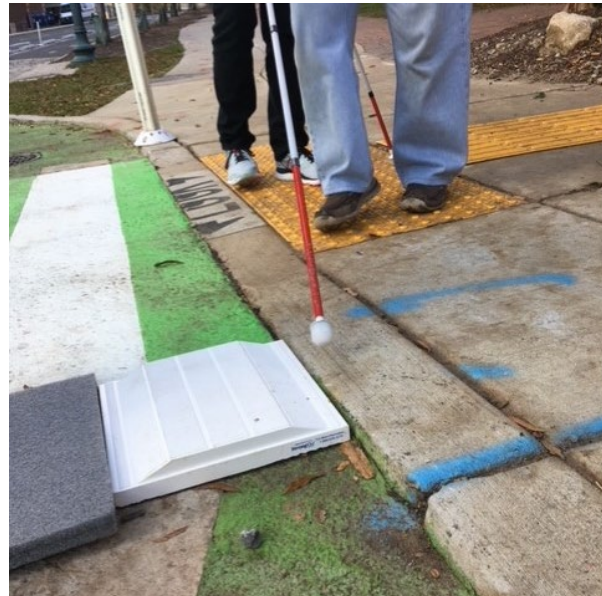
Figure 7: Example of a raised trapezoidal delineator (white raised surface) in Montgomery County
