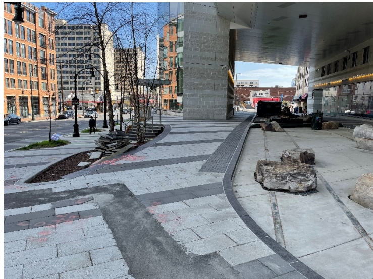
Figure 44: View from Wayne Avenue toward the Fenton Street entrance of the Silver Spring Public Library.
