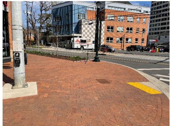
Figure 46: The distance between this APS pushbutton and the top of the curb ramp serving the crosswalk across Bonifant Street is more than 10 feet.
