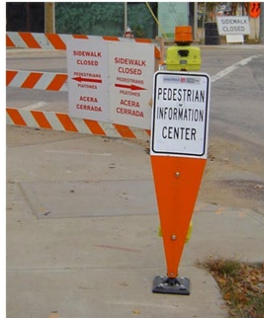
Figure 52: Example of an audible speech messaging device posted in advance of a work zone.
