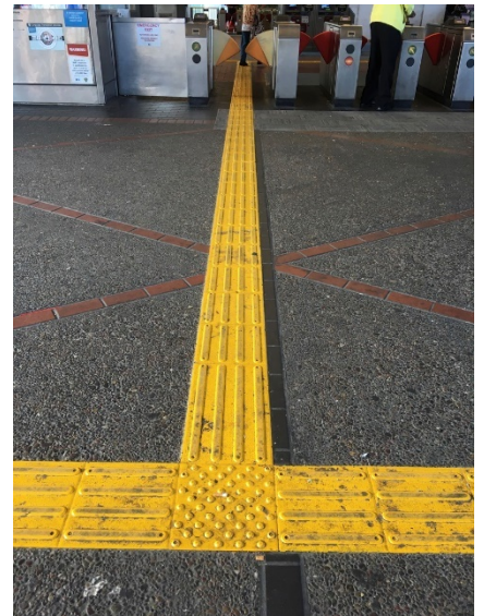
Figure 18: Guidance strips have been installed around the San Francisco Bay Area to help people with vision disabilities locate and navigate through BART transit stations. The images above are from a transit station in Contra Costa County. The indicators begin on the sidewalk about a block away from the station entrance and define a continuous path from the sidewalk, through the turnstiles, to the escalator and ultimately to the platform.
