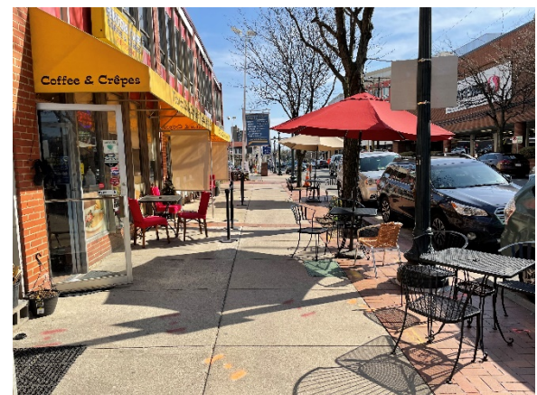
Figure 51: Cafe seating extends into the pedestrian access route on the sidewalk.
