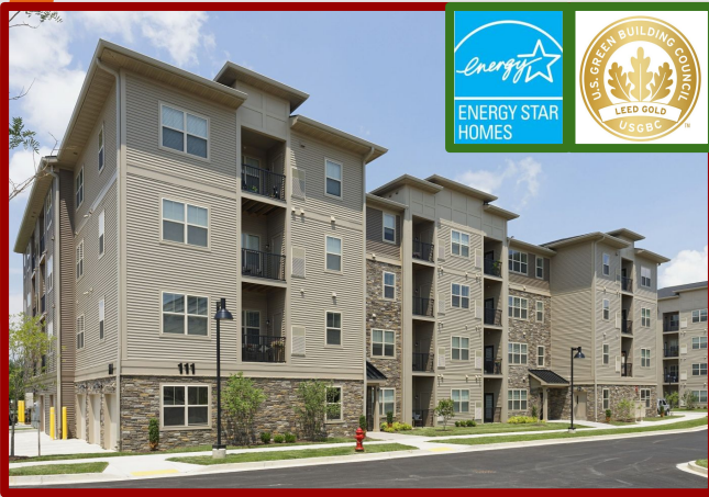
East of Market Apartments
