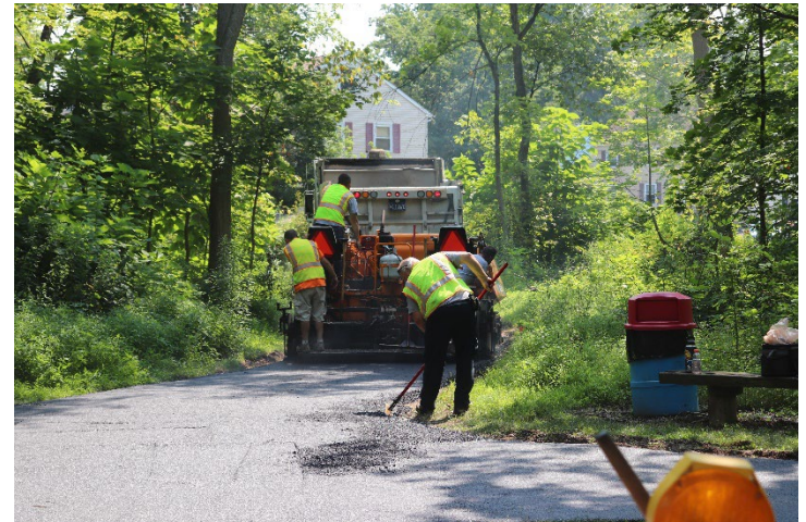
Public Works crew
