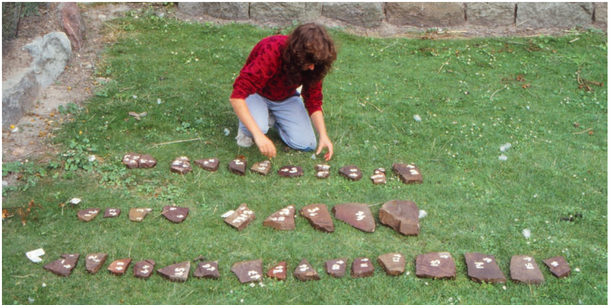
Fig. 3. Flagstones in three sections of dry-walling in the passage grave Kong Svends Høj had to be dismantled. They are seen here after removal, laid out to enable investigations of their working and fitting together (photo: T. Dehn).
