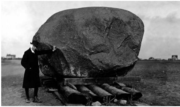
Fig. 7. A 50t erratic having been removed on a wooden sledge in the course of tube construction in Berlin 1912 (BZ online 2013).
