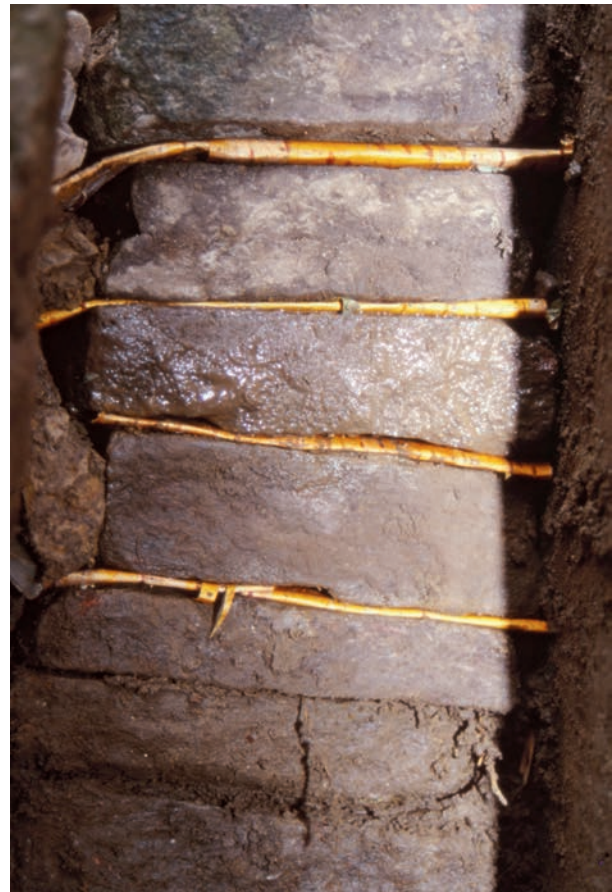
Fig. 2. Section of the rebuilt dry-walling shown on figure 1. Folded, fresh birch bark has been laid between five recently-added sandstone flags (photo: T. Dehn).
