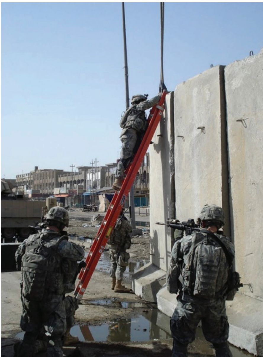
Figure 3. Infantry Soldiers emplace a section of T-wall.
