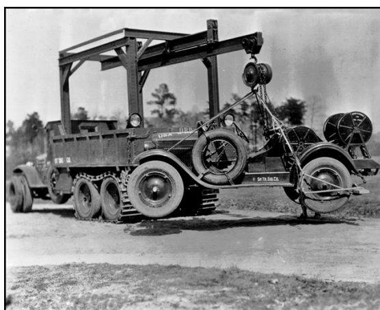
MacArthur's directive was for each branch to experiment with mechanization. Above, a dual-tandem-wheeled crane truck with tracked tires lifts a Signal Corps cable-laying car.
