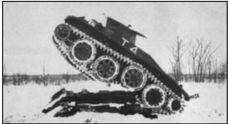
Christie-based Combat Car T-4 climbs log ramp during tests in 1934.
