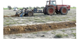
Ripping and mounding
