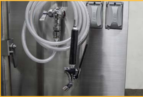
OA-215 - SPRAY RINSE WITH CONTROL VALVE AND VACUUM BREAKER Wall mounted spray rinse hose assembly.
