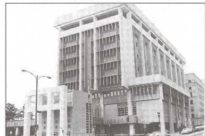
District One Police Administration Building 951 N. James Lovell Street, Milwaukee, WI 53233
