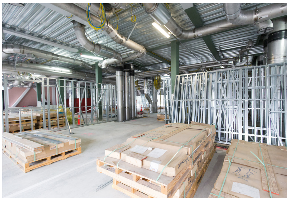
Figure 2: First-floor steel wall framing and above-ceiling heating, ventilation and air-conditioning system
