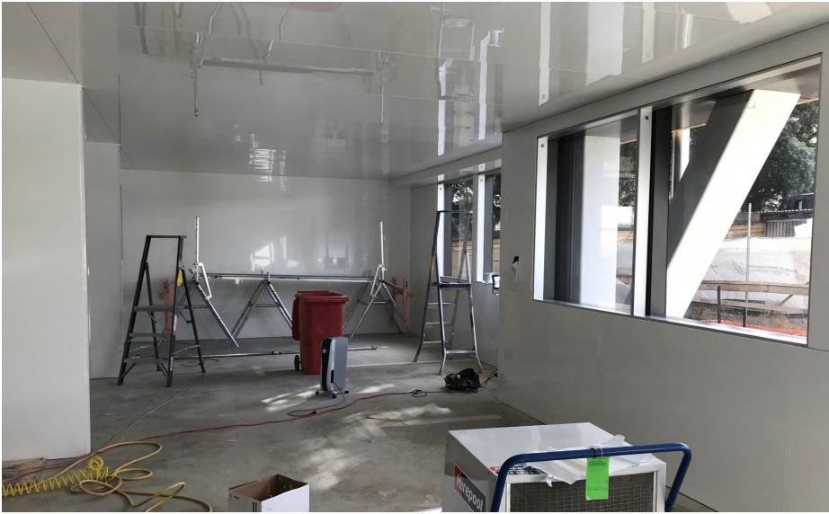
Figure 3: A ground-floor laboratory showing smooth high-gloss Arcoplast panels that are resistant to impact, corrosion and chemicals
