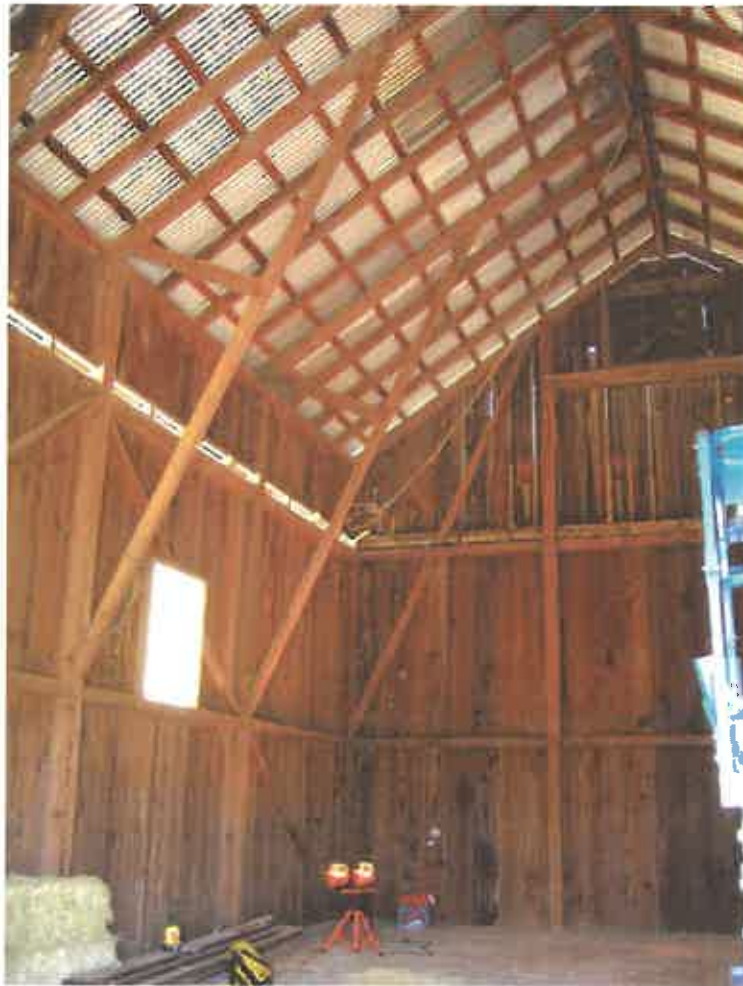
Figure 25. Wall and roof framing systems at the center aisle.
