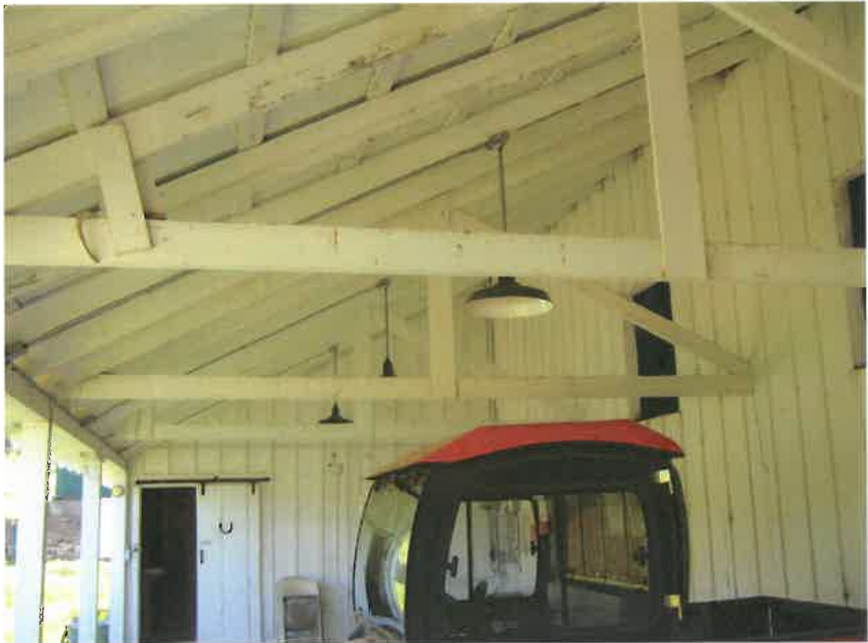
Figure 32. Roof framing system at the east aisle.
