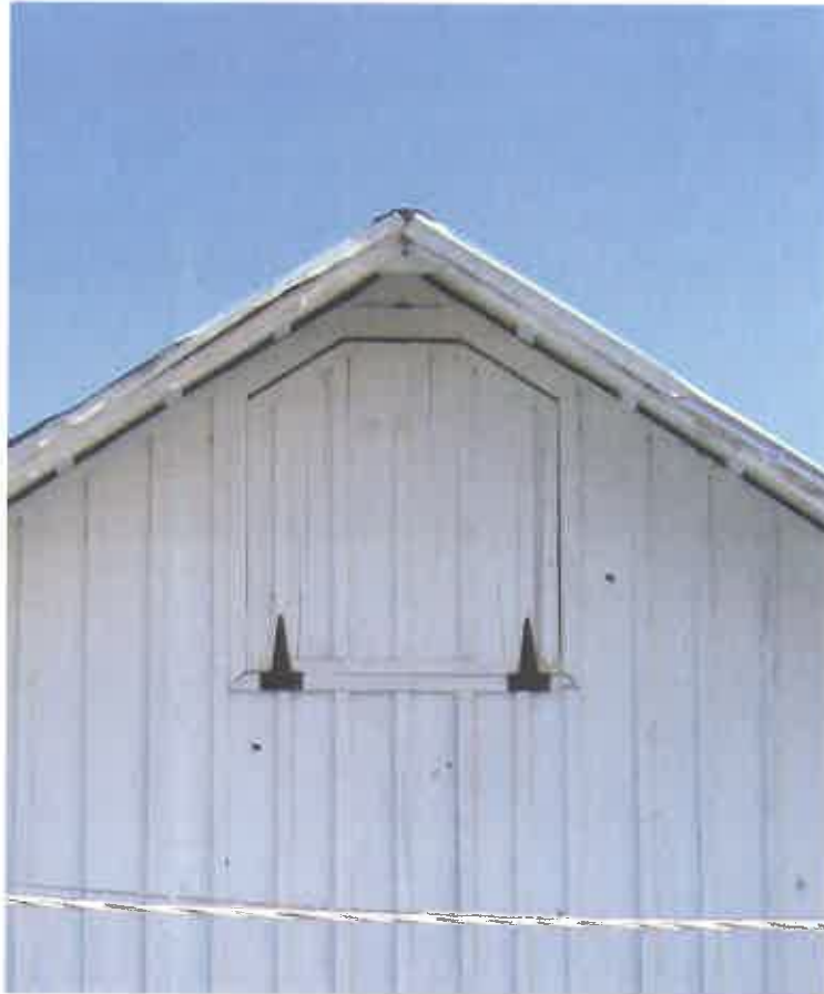
Figure 21. Hay loft door at the south elevation.
