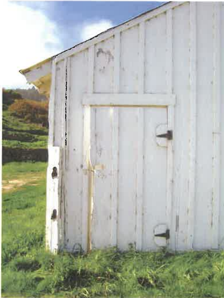
Figure 15. Hinged door leading to the east aisle.
