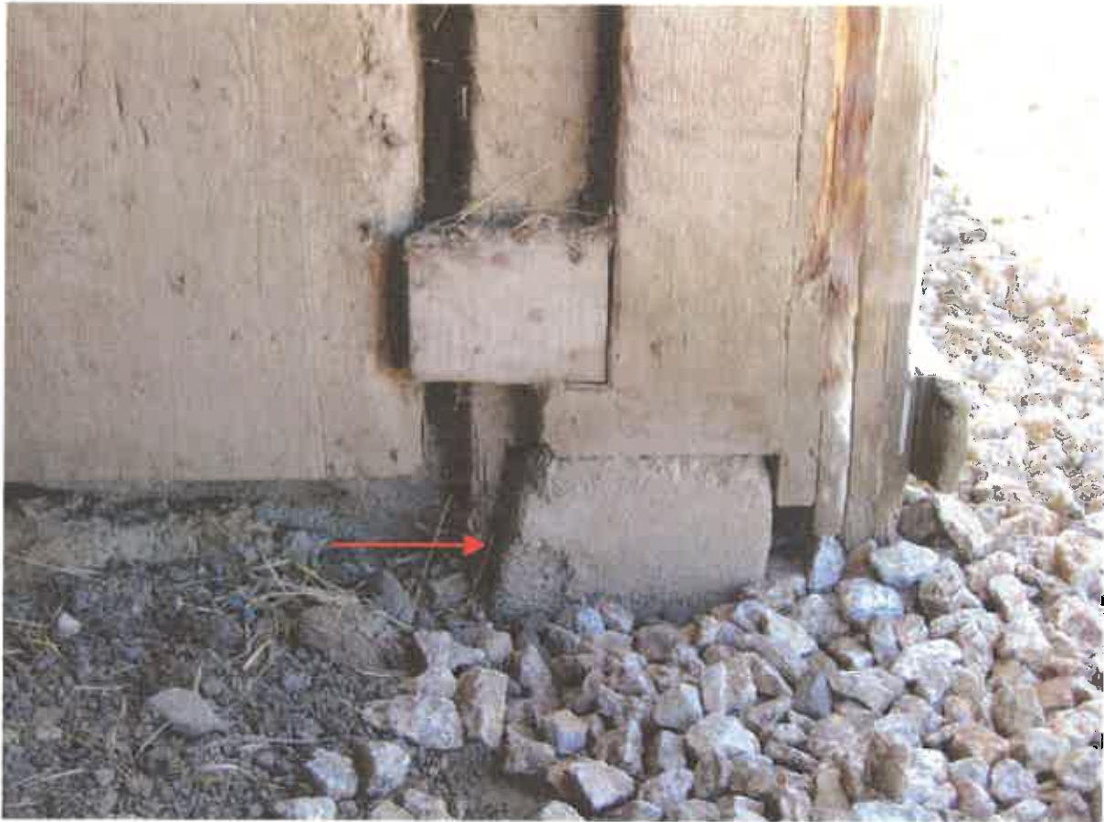
Figure 45. Subgrade perimeter foundation at the west elevation.
