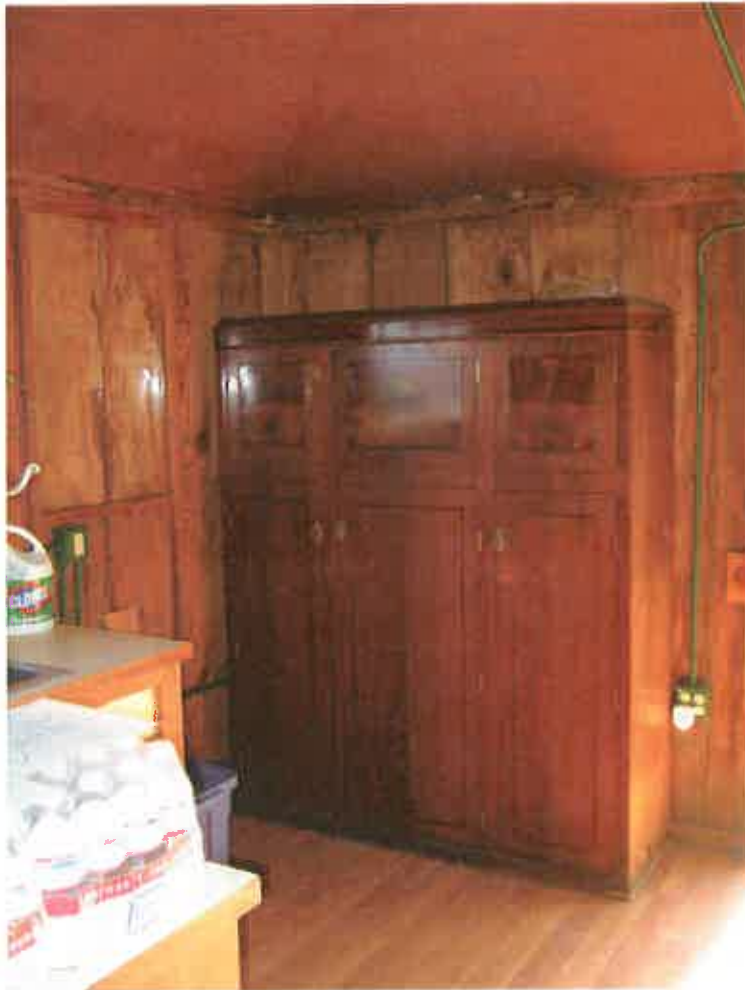
Figure 38. Cabinet located in the southeast corner of the kitchen.
