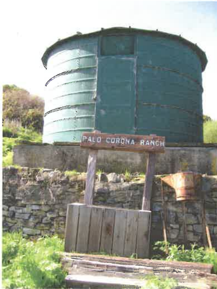
Figure 43. Silo sitting on top of the stone retaining wall.
