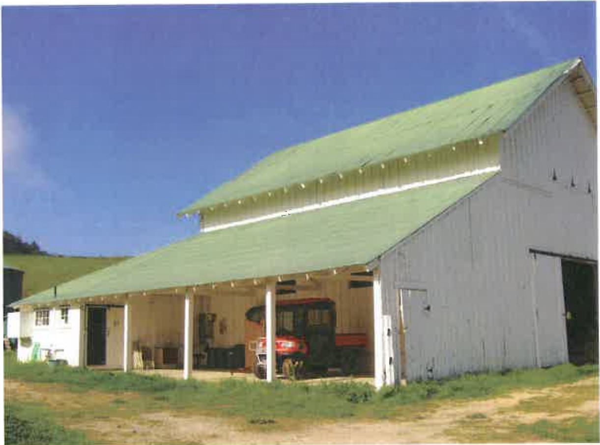
Figure 16. East elevation showing the open-sided east aisle and rear storage area.
