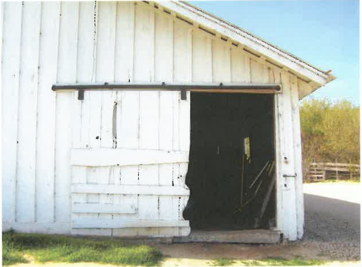
Figure 14. Sliding barn door at the north elevation leading to the west aisle horse stalls.
