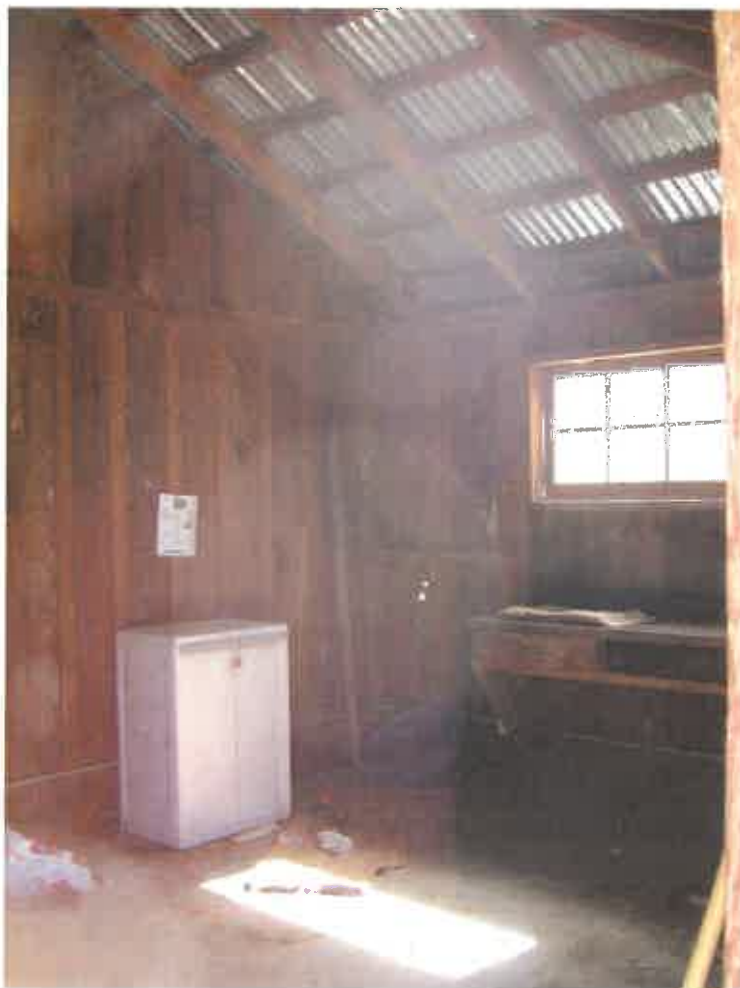
Figure 41. Rear storage room #3.
