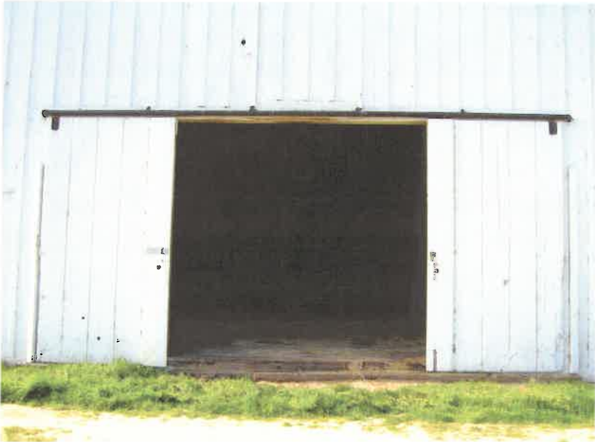
Figure 13. Sliding barn doors at the north elevation leading to the center aisle.
