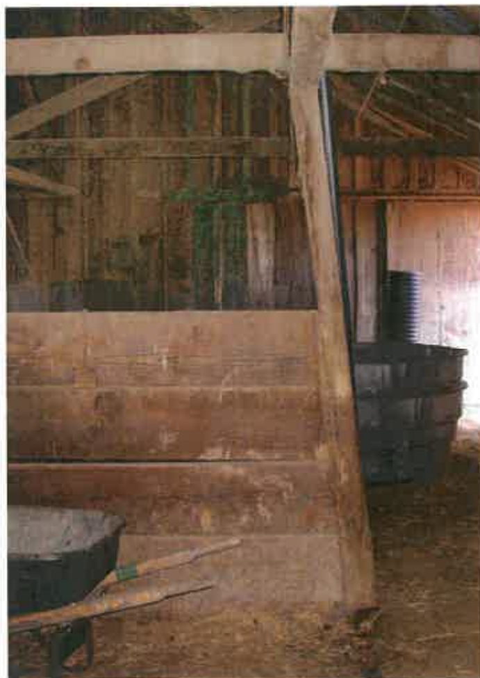
Figure 30. Dividing horse stall wall at the west aisle.
