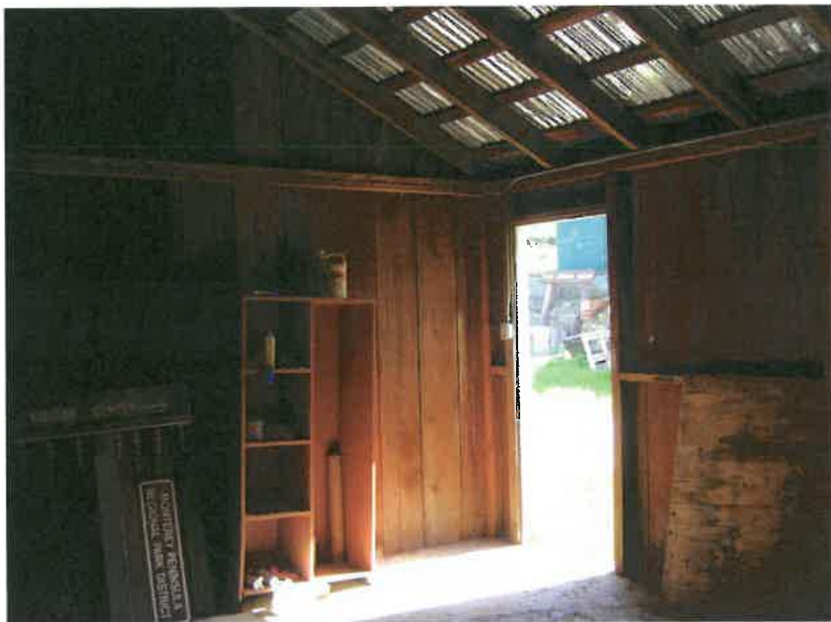
Figure 40. Rear storage room #2.
