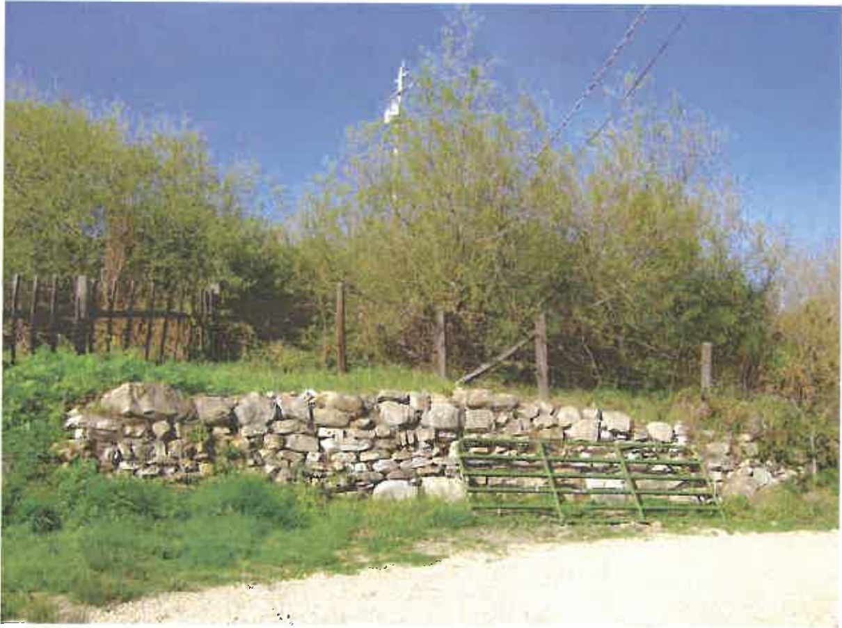
Figure 7. Stone retaining wall located at the south of the barn .
