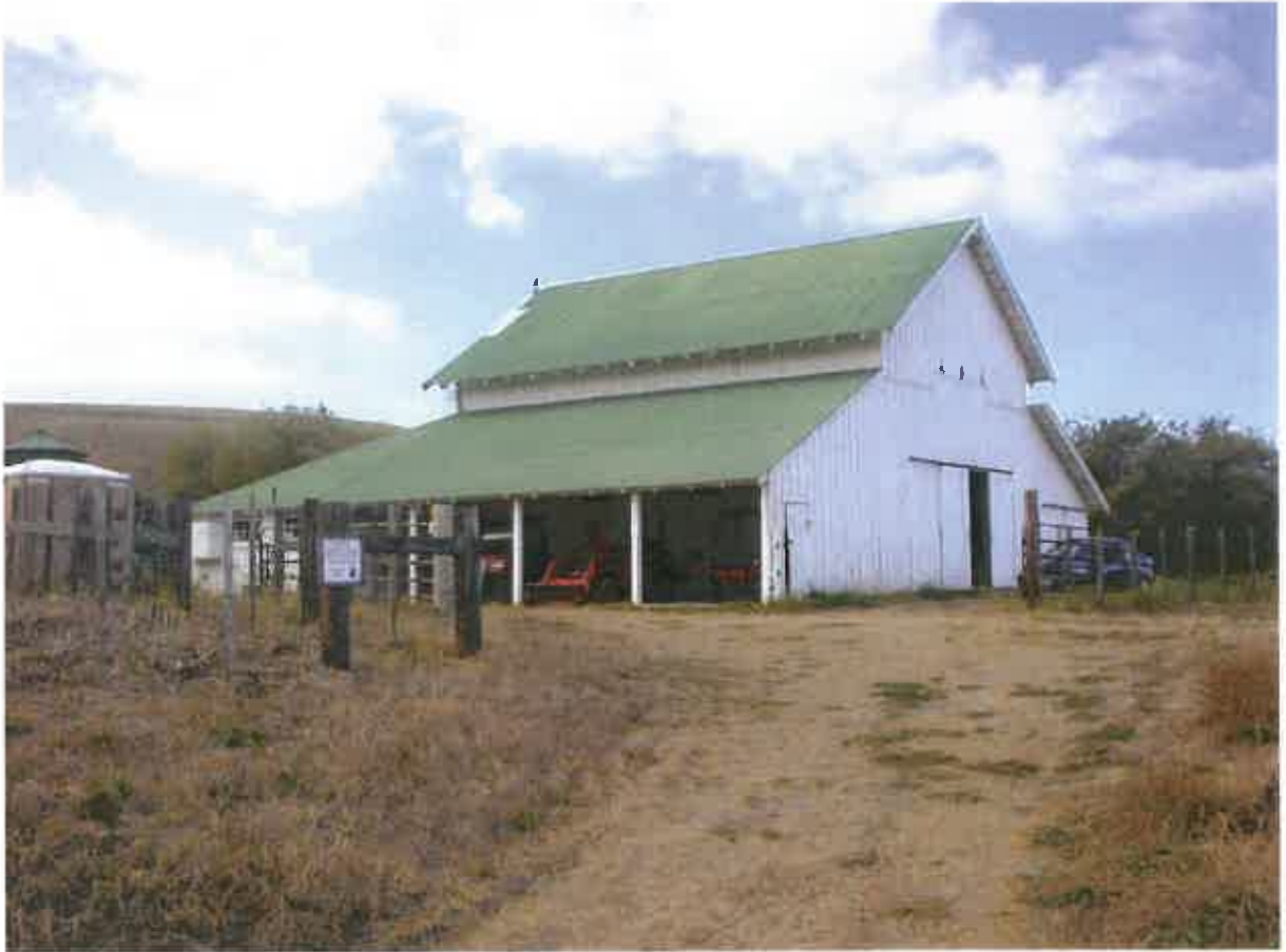
Figure 10. Overall view of the Fish Lower Barn from the east.
