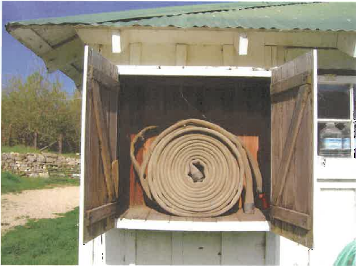
Figure 19. Fire hose located in a cabinet on the east elevation.
