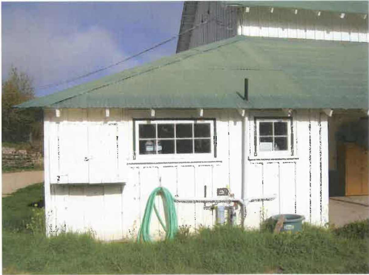
Figure 18. Windows at the east elevation of the rear storage area.
