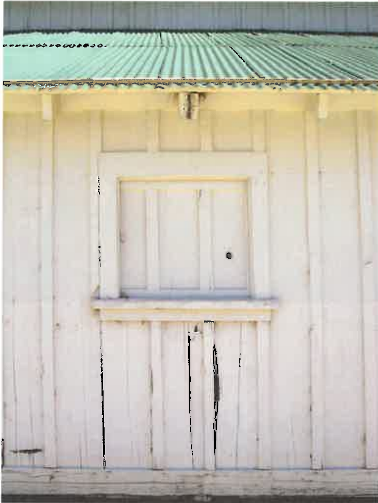
Figure 23. Typical sliding window at the west elevation.
