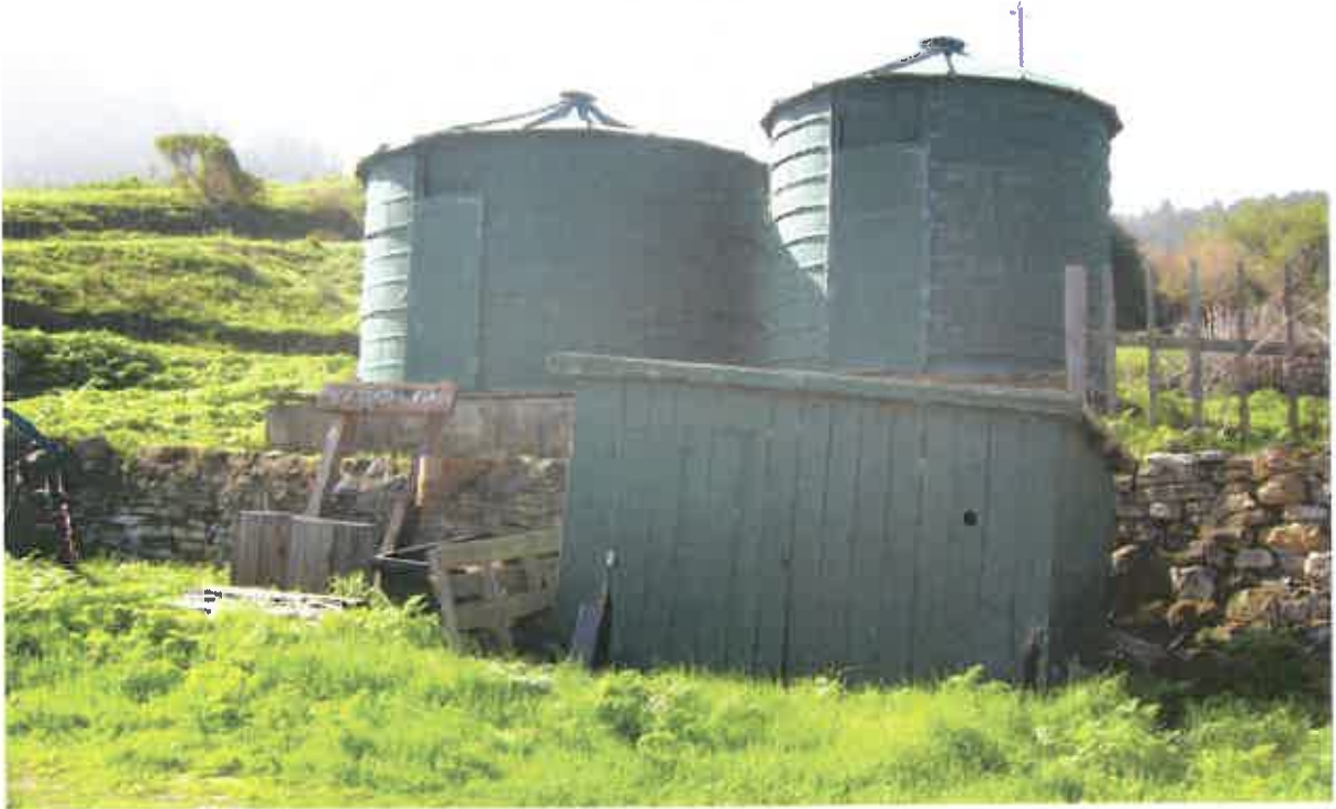
Figure 8. Silos sitting on top of the eastern portion of the retaining wall. Small shed, sign, and other ranch equipment leaning against wall.
