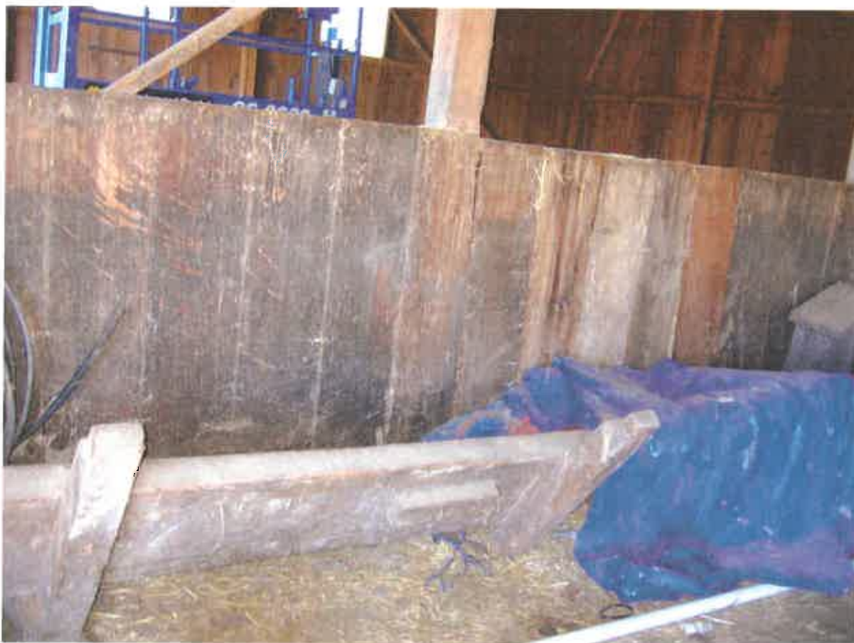
Figure 31. Horse trough along the lower east wall in the west aisle.
