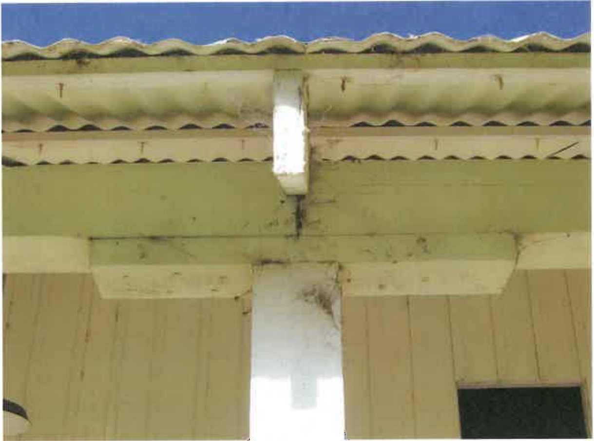
Figure 34. Structural framing system of the east aisle.
