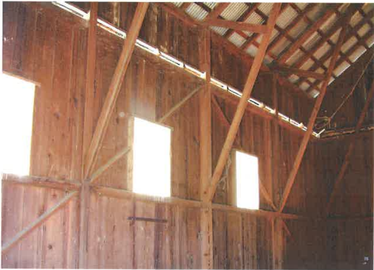
Figure 29. Openings at the east interior elevation wall in the center aisle.
