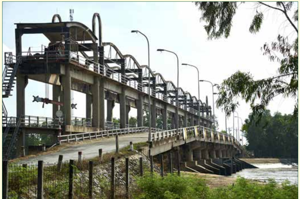
Sluice gates across the Ba Lai River in the maritime Vietnamese province of Ben Tre. The gates can be used to stop saltwater intrusion into Mekong Delta farmlands that rely on freshwater. Ben Tre is a leading producer of coconuts.
