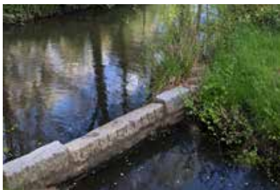
Image 64: Billabong Chain granite weir.
