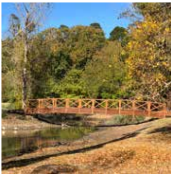
Image 13. New Bridge dominates landscape, island in poor condition
