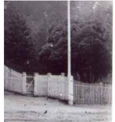
Image 49 Detail showing the c. 1913 timber gate and arrangement with adjacent timber picket fence along Mollison street.
