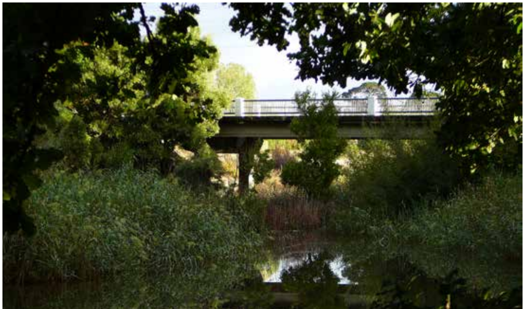
Image 55. Coliban River Bridge Malmsbury n.d. Malmsbury Historical Society
