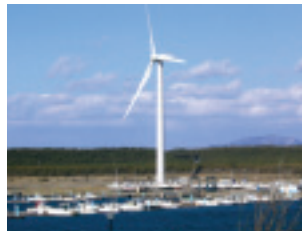
An NPO-operated community wind turbine in Akita City
