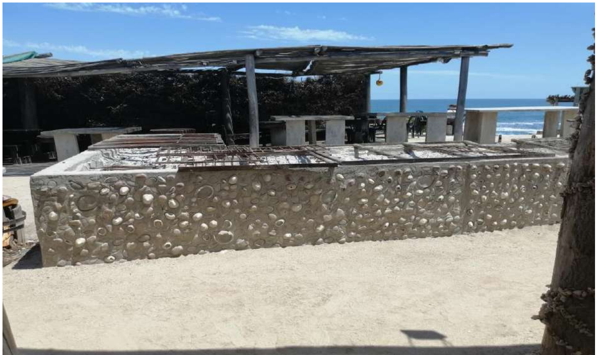
Photo 2: The fire place inside the wooden structure
