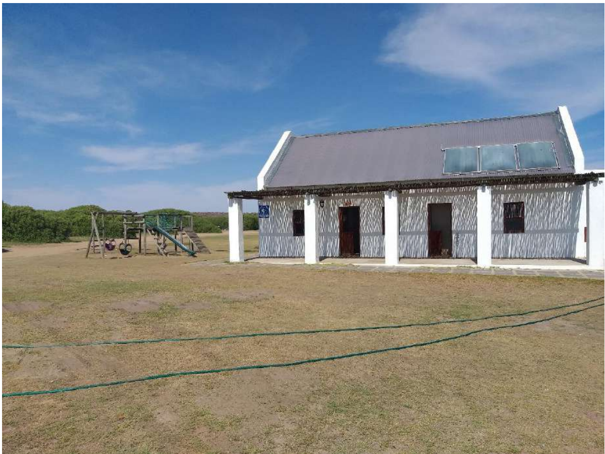
Detail view of the northern elevation of an ablution facility.
