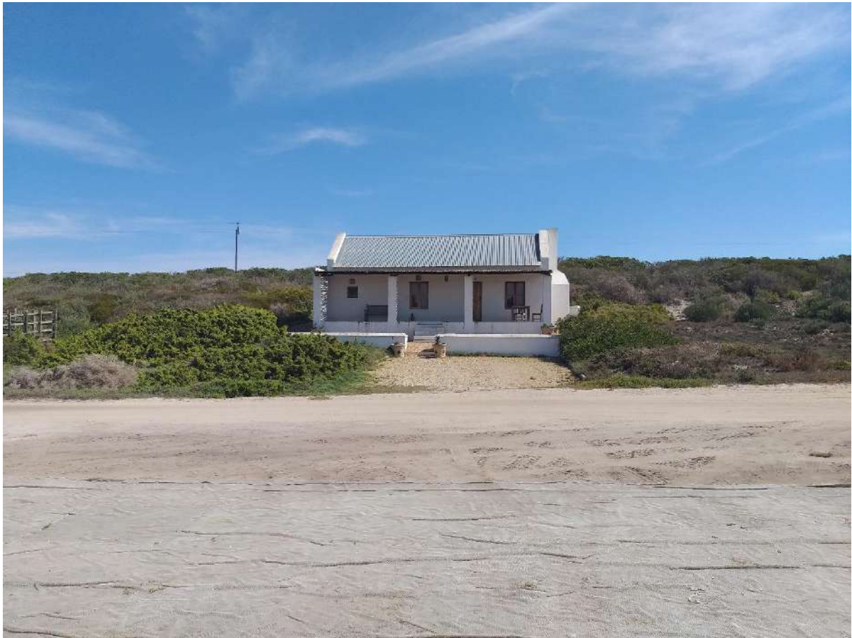
Malkoppan view of the old existing cottage that was refurbished for accommodation.
