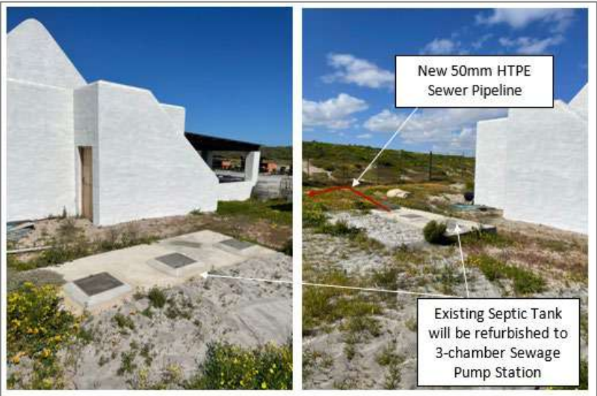
Figure 3. Pump Station 2 (Malkoppan Recreational Building/Brouery) and Pipeline
