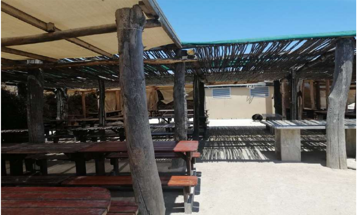
Photo 3: Inside of the wooden structure
