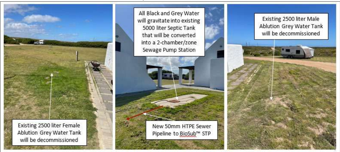
Figure 5. Pump Station 4 (Malkoppan Main Campsite Male and Female Ablutions)
