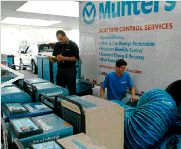
Day 1 10:30 a.m. | Suitable equipment is prepared at Munters' service depot ▶
