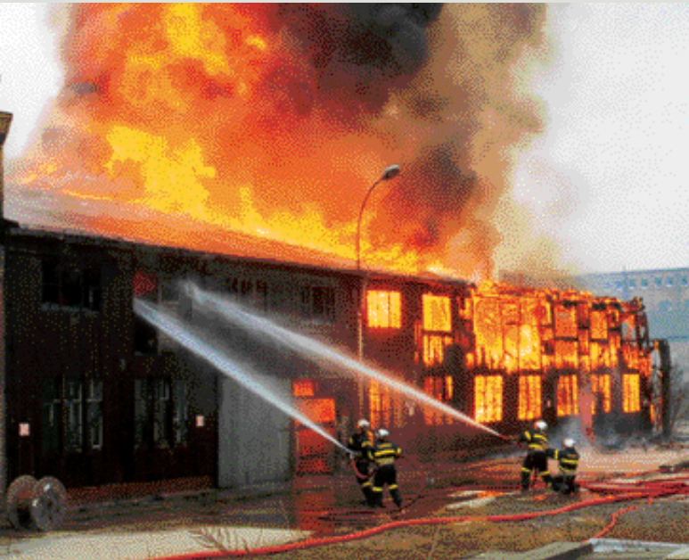
Day 1 09:00 a.m. | A building is damaged
