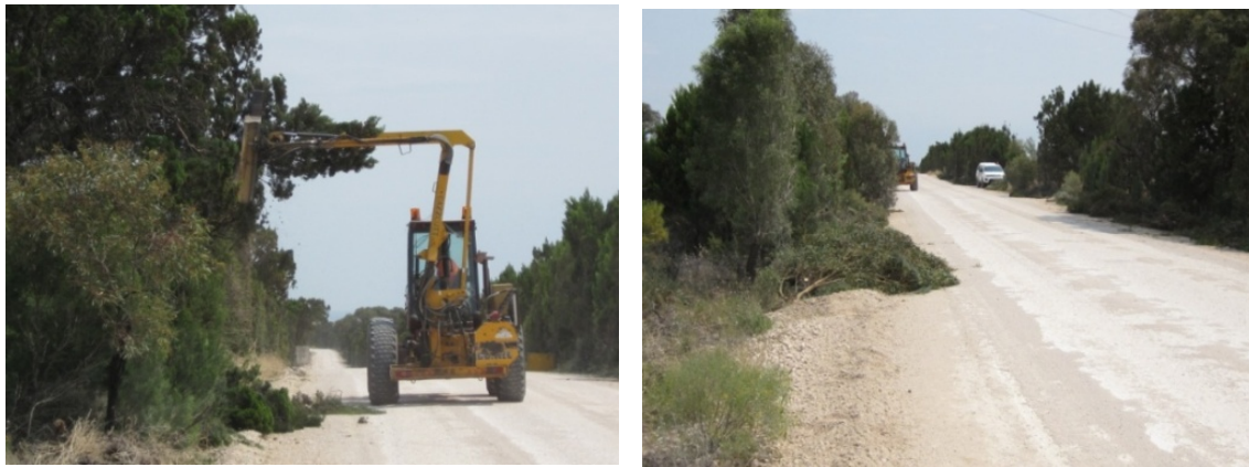
Figure 22: Vegetative management by cutting with a saw and slashing prunings on the ground
