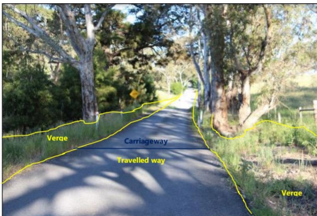
Figure 21: Verge is directly adjacent to the bitumen, and regrowth clearance is restricted to understorey only in this instance. The large trees would not fall under these guidelines and clearance would require an application, as they are not considered regrowth.
