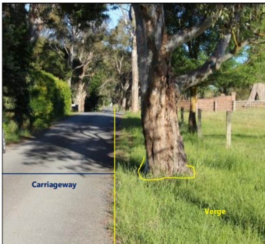
Figure 19: Travelled way and carriageway are the same widths in this instance, with verge regrowth clearance restricted to understorey only.
