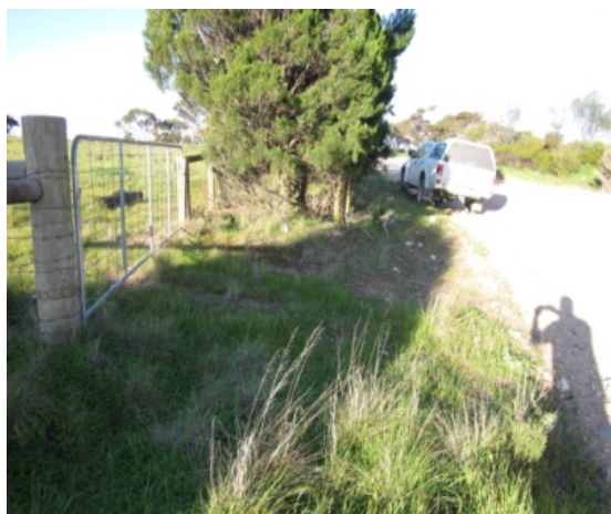
Figure 28: Poor Driveway sight clearance
