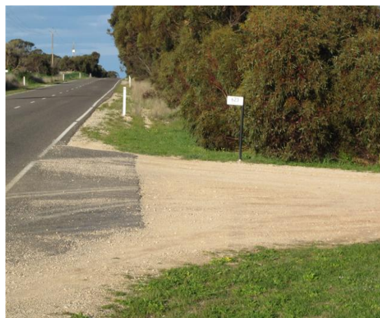
Good driveway sight clearance
