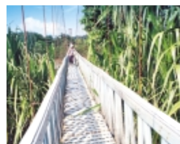
The Company used recycled plastic to construct this pedestrian bridge in Costa Rica.
