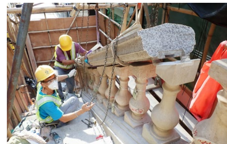
28 工匠利用鏈條起重器及手動工具進行構件重組工程 Artisans used chain hoists and hand tools during the reinstallation works.
