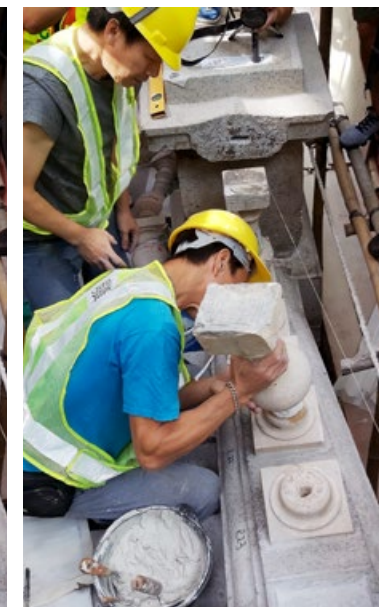
28 工匠利用鏈條起重器及手動工具進行構件重組工程 Artisans used chain hoists and hand tools during the reinstallation works.
