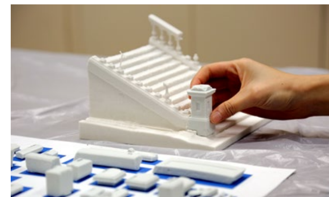
23 工程人員透過三維打印技術製成花崗石碎片微縮模型，並標示號碼，在工作室將破損古蹟組合。 Miniature replicas of the numbered granite fragments were 3D-printed and reassembled in AMO office.
