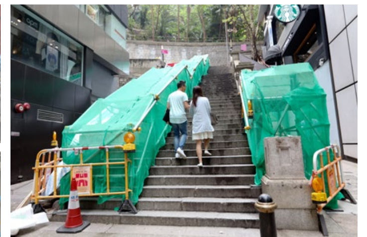
11 石階完成結構安全評估及架設臨時防護圍欄後，局部重開。 The steps were partially reopened after their structural safety had been confirmed and temporary protective fencing had been erected.
