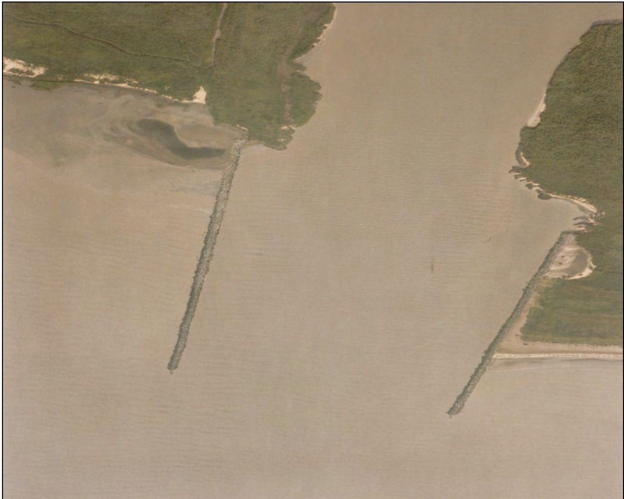
Mermentau River Shoreline BU Placement Site (13 August 1991)
