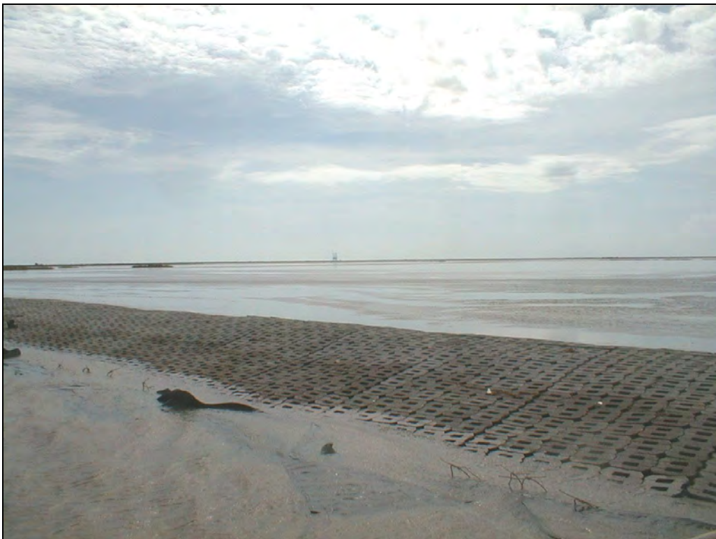
Lower Mud Lake BU Placement Cell: ACM Protection (21 November 2000)
