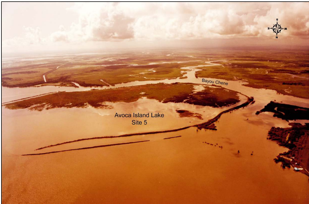
Avoca Island Lake Disposal Site 5 - 1981
