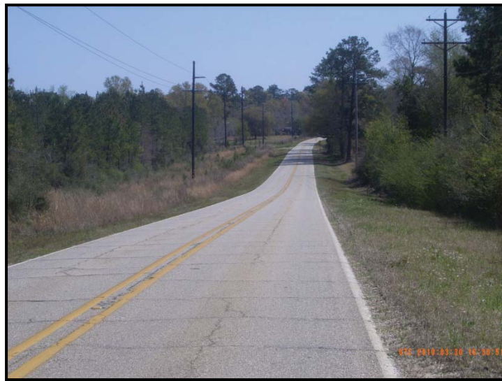
Figure 3-20. LA 435: Looking westbound near Talisheek.
