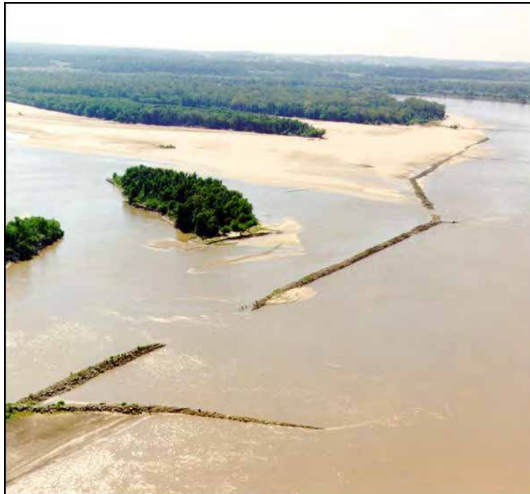
Photograph 7-3. L-Head Dike, Marquette Chute, near Middle Mississippi River Mile 51.0L
