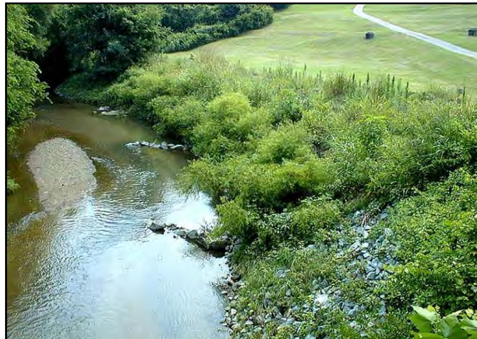
Photograph 7-21. Rock Vanes with Bioengineering, Urban Setting, Charlotte, NC (photograph: Andrew Burg)
