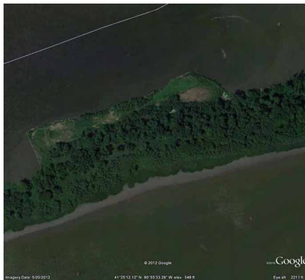
Photograph 7- 13. Hershey Chute Rock Revetment, River Mile 461.5, circa 2012
