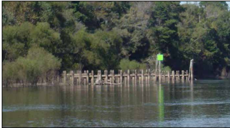
Photograph 7-23. Permeable Wooden Pile Dike on the Apalachicola River, FL
