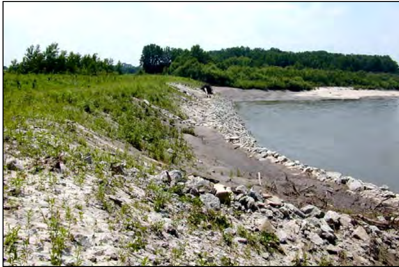
Photograph 7-20. Longitudinal Peak Stone Toe Protection
