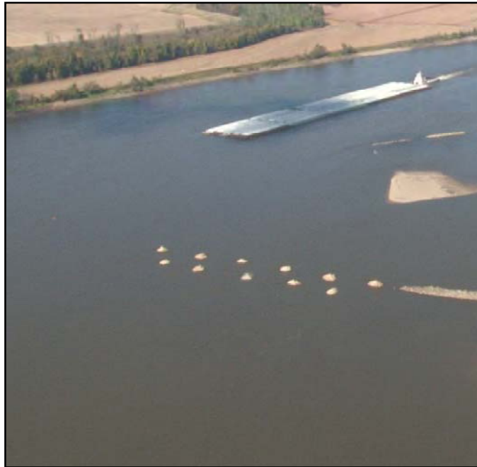
Photograph 7-18. US Army Corps of Engineers, St. Louis District Riprap Landing Multiple Roundpoint Structures, Middle Mississippi River Mile 265.7.
