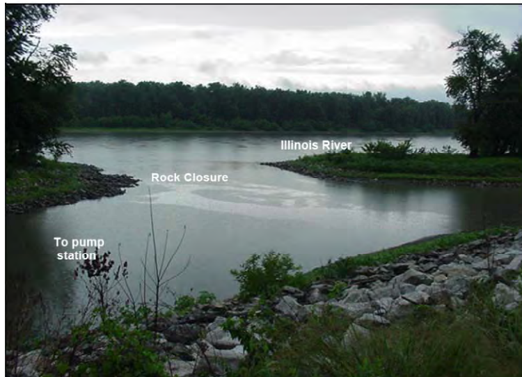
Photograph 7-2. Submerged Rock Closure Structure at Liverpool Ditch, Illinois River (August 2004)
