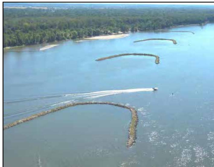
Photograph 7-8. A Series of Chevrons Aligned To Split Flow Between the Main Channel and a Side Channel, While Protecting the Existing Shoreline
