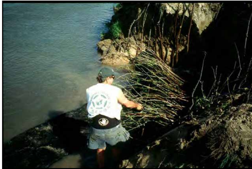
Photograph 7-22. Bioengineering Using Willow
