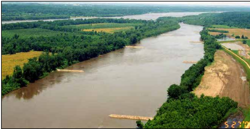
Photograph 7-6. Santa Fe Chute Alternating Dikes
