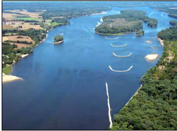
Photograph 7-7. A Series of Chevron Dikes on the Mississippi River
