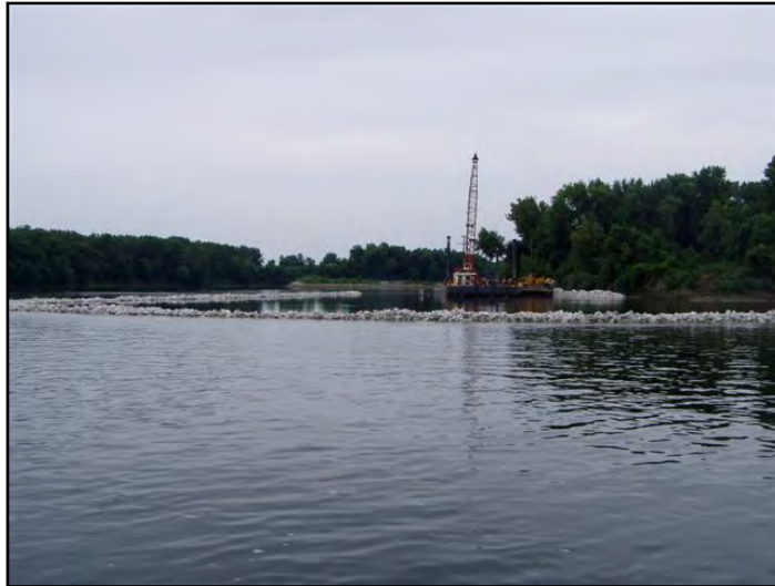
Photograph 7-11. LaGrange Island Bluntnose Chevron Rock Placement, Looking South East – August 2005
