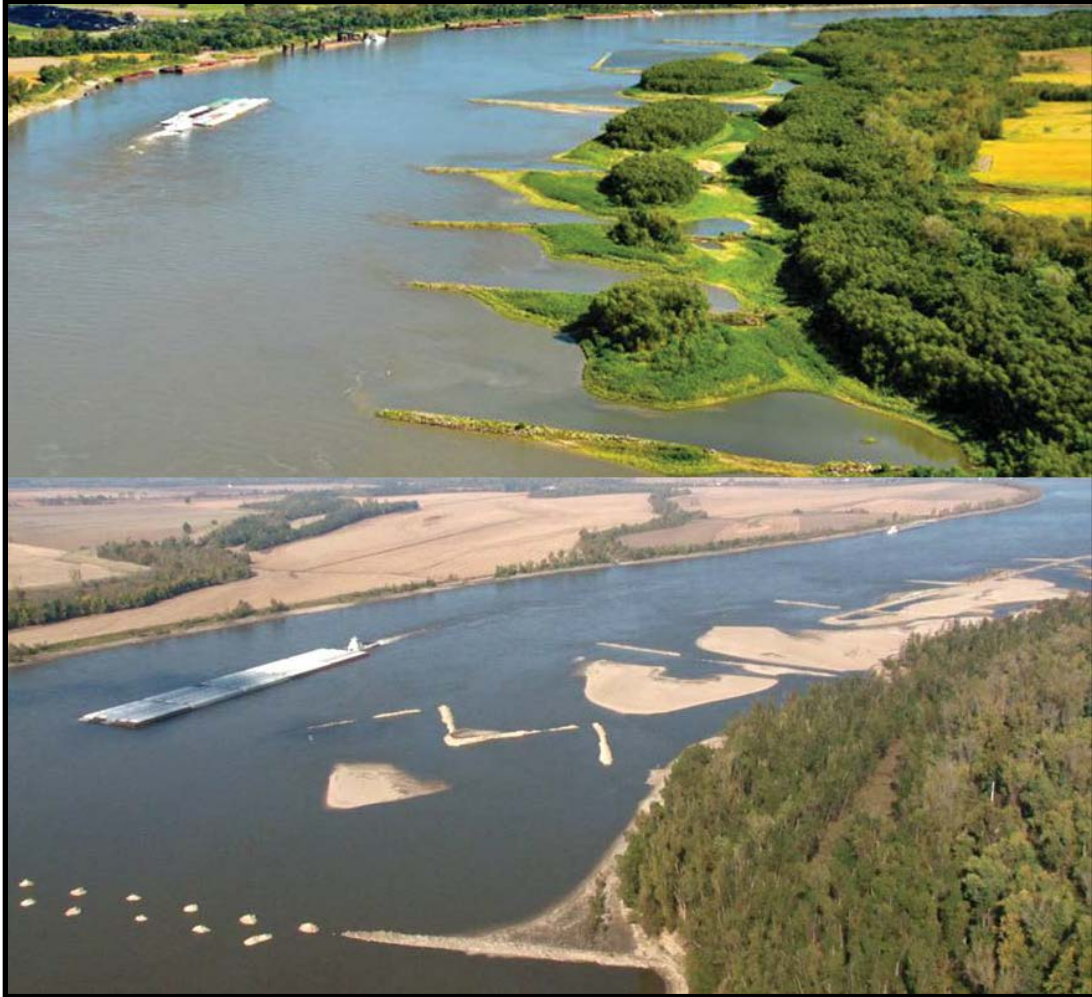
Figure 2. Examples of river training structures on the Middle Mississippi River.
