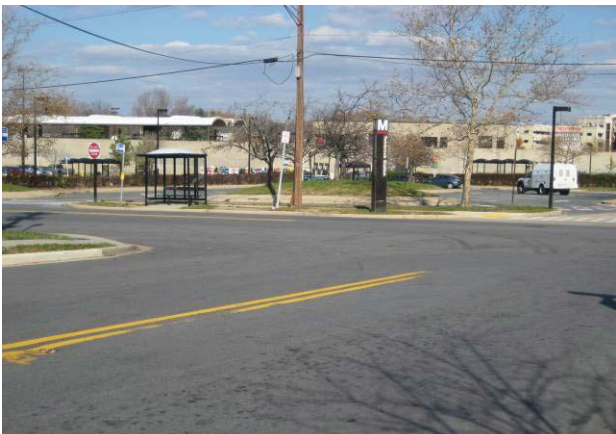
Missing crosswalks at Metro station entrance on Chapman Avenue
