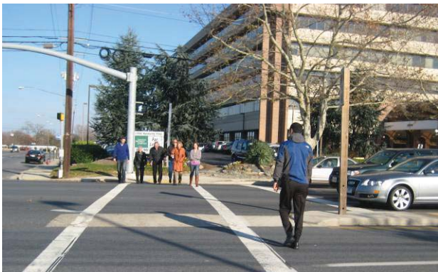
Unprotected at-grade median
