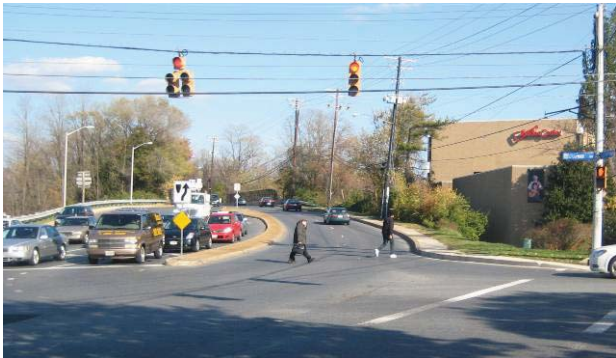
Missing crosswalks at Chapman Avenue and east side of Twinbrook Parkway
