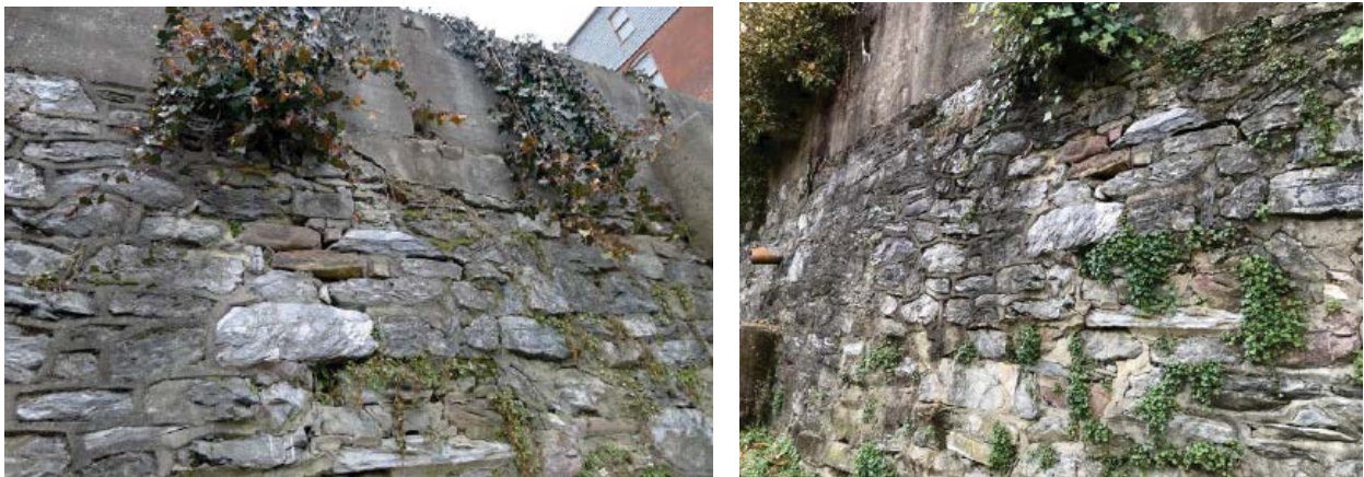
Photograph 2. Floodwall Repairs near Market St. Bridge (Alternative 2.B)
