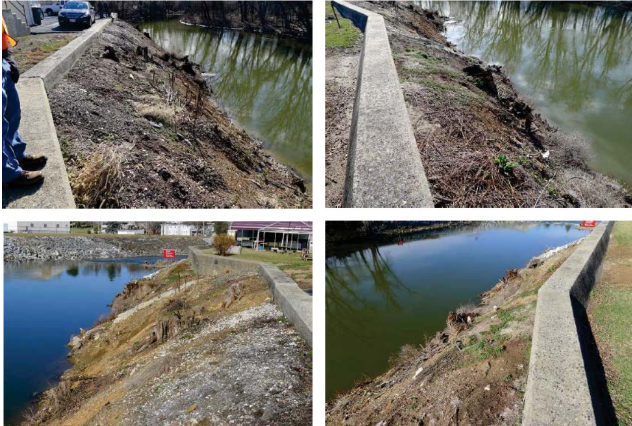
Photograph 3. Riprap Installation near S. Richland Ave. Bridge (Alternative 2.C)
