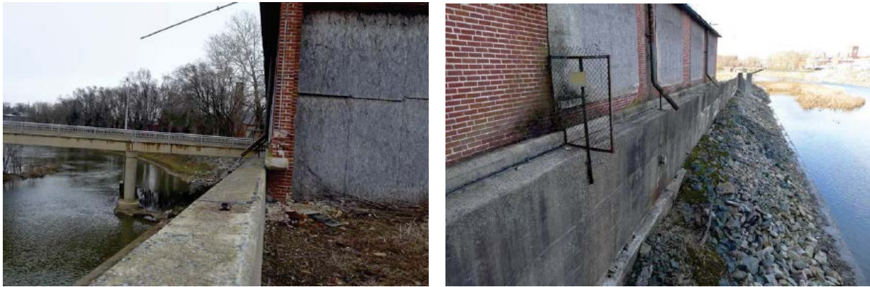
Photograph 1. Floodwall Replacement near Penn St. Bridge (Alternative 2.A)
