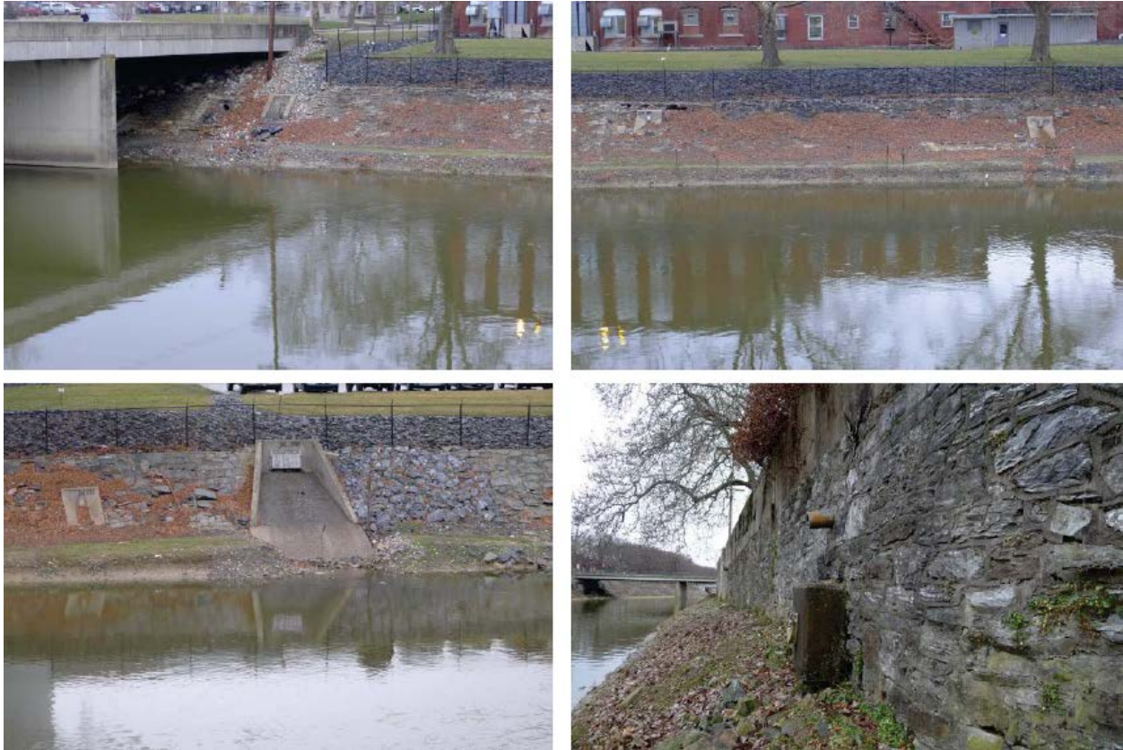
Photograph 4. Examples of Drainage Conduit Maintenance (Alternative 2.D)
