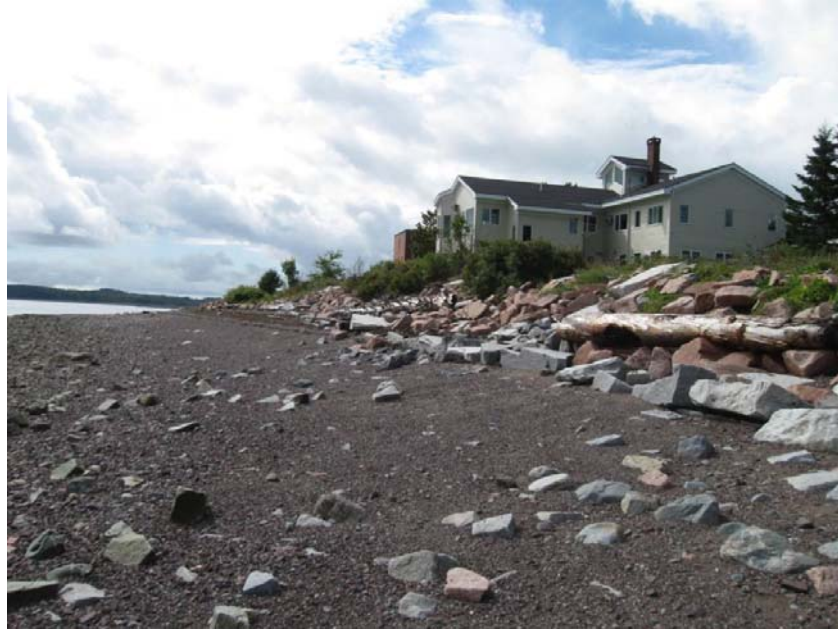
Figure 3 - Area along proposed revetment
