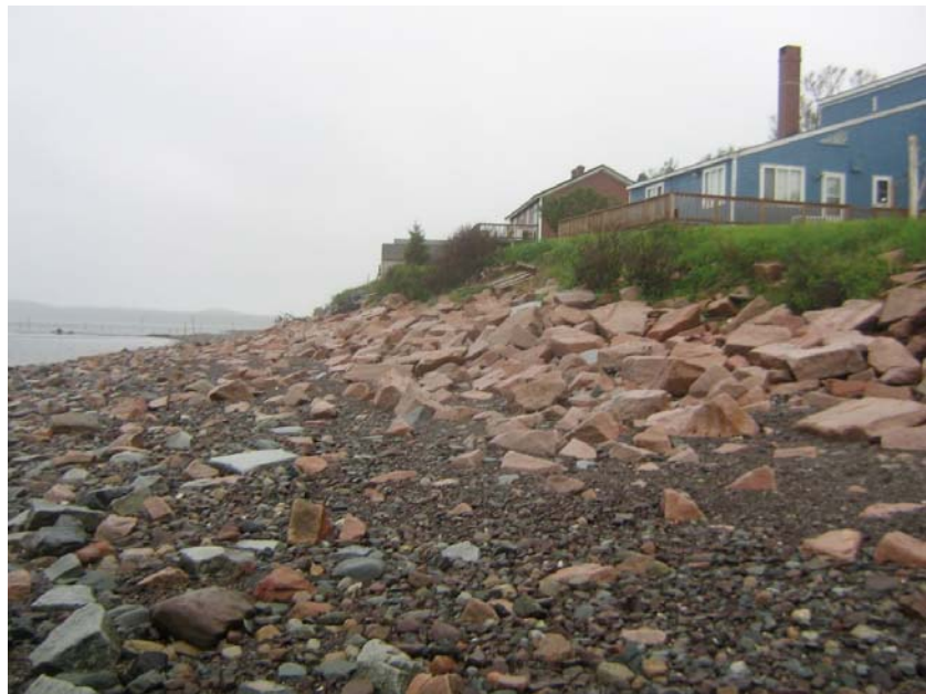
Figure 4 - Looking south in the area for the proposed revetment
