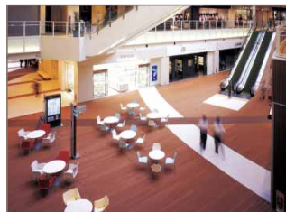
Pluswood, a composite material made from wood powder and non-vinyl chloride thermoplastic
