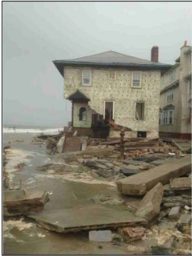
Damage to house in Brooklyn, NY (Proud Novice, 30 Oct 2012)
