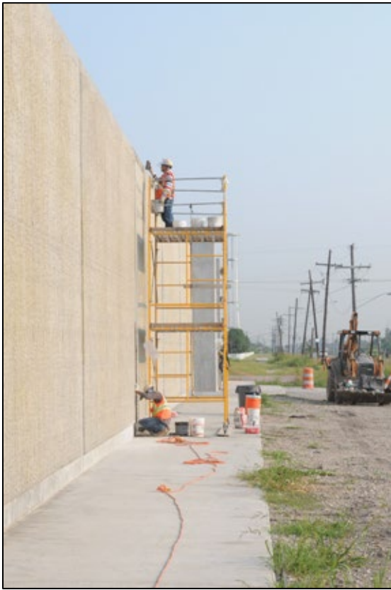
Figure 28: Floodwall under construction in New Orleans, LA.
