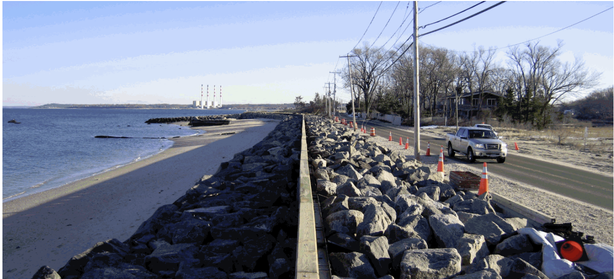
Figure 3 Repaired/Modified 103 Project (Reach 1a)
