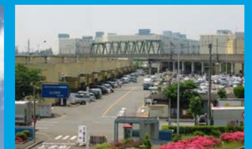
Osaka Prefectural Food Distribution Center
