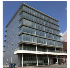
Nankai Wakayamashi Station office building
