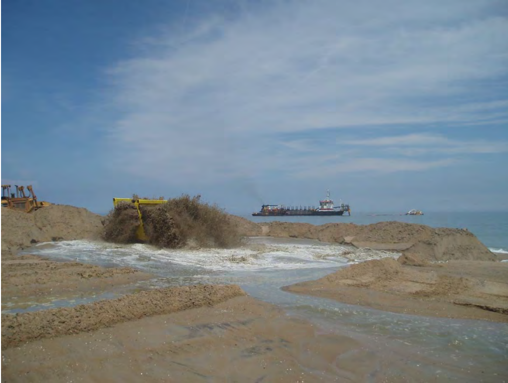
Figure 3-4. Sand Being Pumped Through a 3/4 -inch MEC Screen Basket from a Hopper Dredge. (background). Training berms surround pump-out area to allow for sand to settle out.
