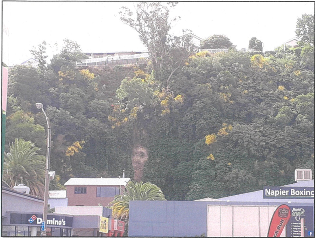
Photo 5: Cut Slope above Craven Terrace
