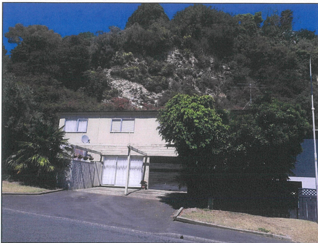
Photo 7: Cut Slope above lower Burns Road
