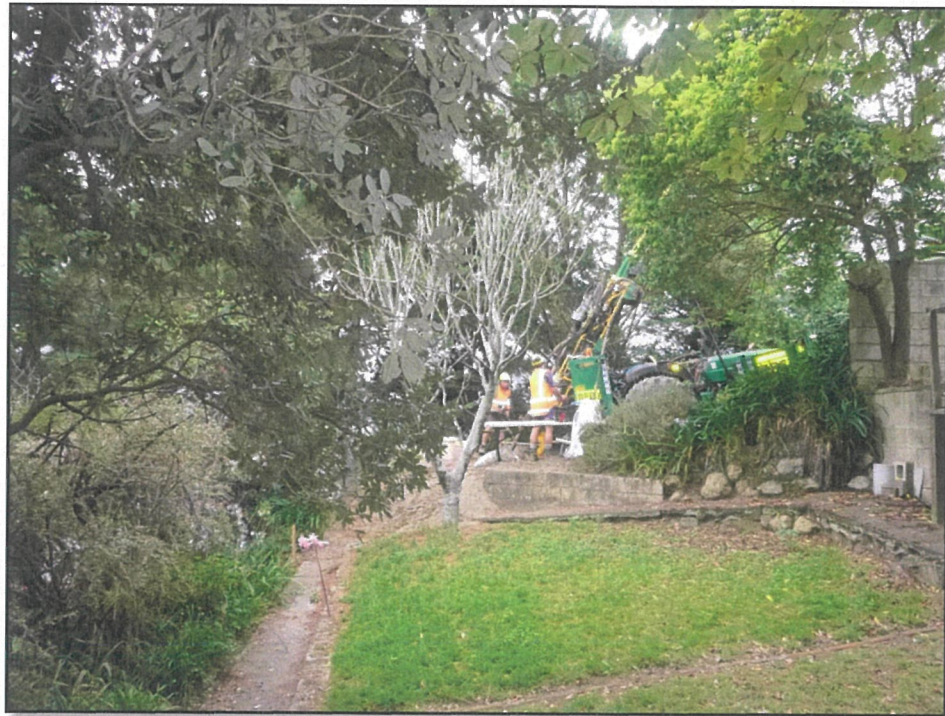
Photo 4: Drilling Rig set up at top of existing hill slope
