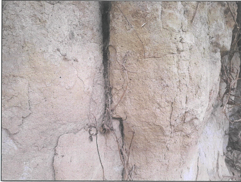
Photo 2: Natural jointing in Loess forming weak columnar structure
