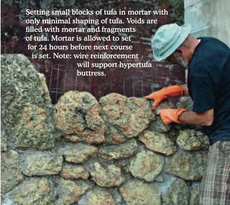
Wire-hypertufa buttresses for added stability. This may not have been necessary.
