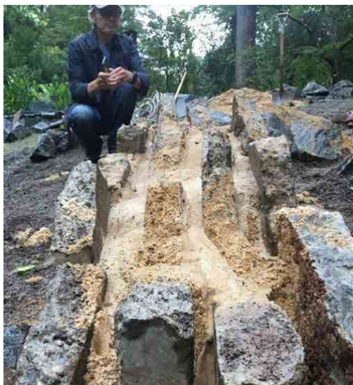
Ozzie Johnson inspecting as the soil mix goes in.
