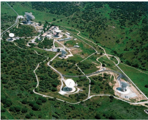
An aerial view of Madrid Deep Space Network Complex.
