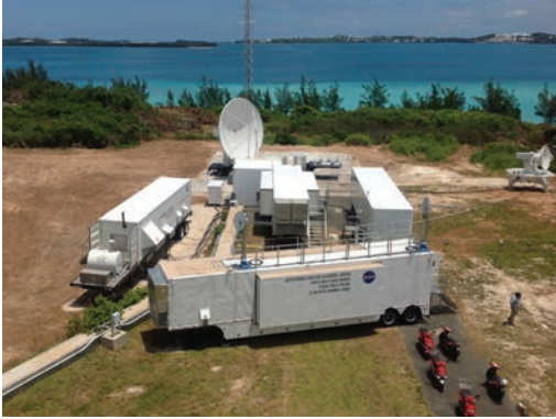
NASA's mobile tracking station in Bermuda provides telemetry, radar, and command and control services.
