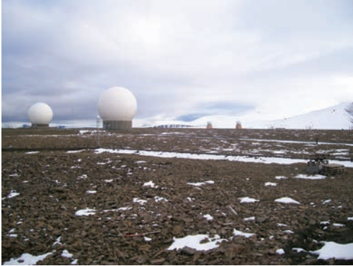
Four of the six protective radar domes (radomes) over the telemetry and command antennas at SvalSat.
