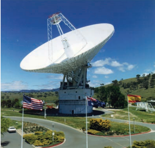
A view of Canberra's 70-meter (230-foot) antenna with flags from the three Deep Space Network sites.
