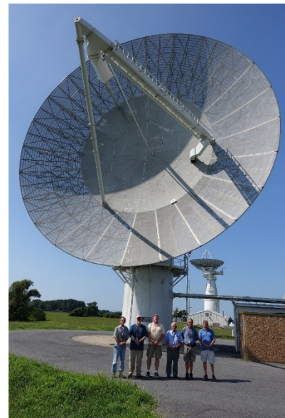
Figure 11.16: 18-meter UHF ground station antenna at NASA Wallops Flight Facility. Credit: NASA.
