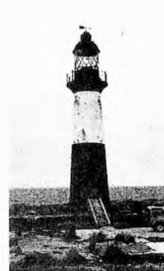
Left: Cape Pembroke Lighthouse before HBC's intervention Right: And after Bottom left: Cartmell Cottage, gifted to the Islands by Nutt Cartmell, being stripped for essential repairs Below centre: The finished article in pristine shape Below right: The German Camp in an unattractive condition Bottom right: The same building after renovation
