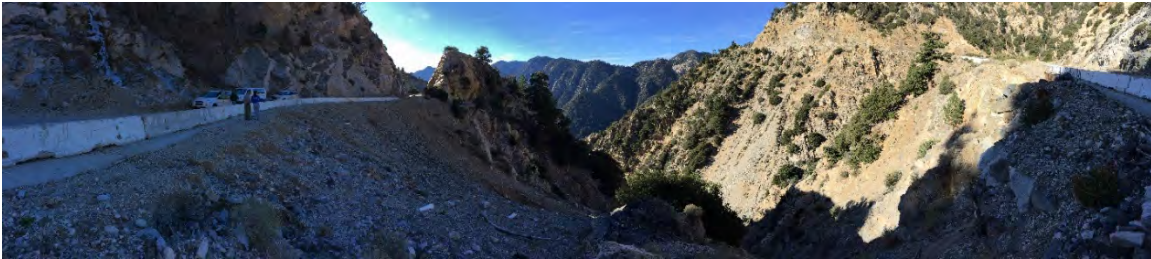
Figure 11. Closed portion of Hwy 39 south of Hwy 2, just west of Mt Islip
