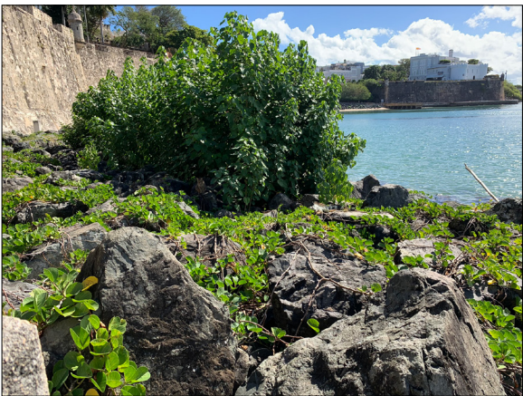
Vines and shrubs grow among the riprap adjacent to the Paseo.
