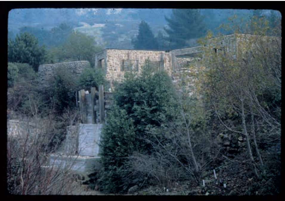
Original visitor center designed by Jim Roof under construction by the garden staff in 1963. This structure was removed and later replaced with the current building.
