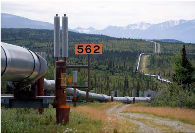
The trans-Alaska pipeline carries oil 800 miles from Prudhoe Bay to the Valdez terminal, in Prince William Sound. Portions of the pipeline are elevated, and refrigerated, to prevent thawing the underlying permafrost. Photo by Luca Galuzzi.
