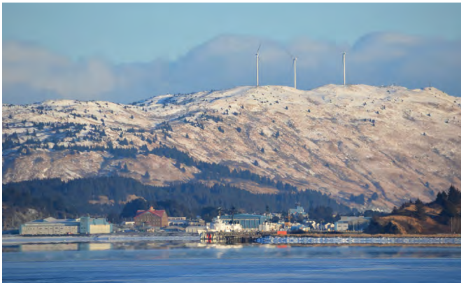
Wind turbines atop Pillar Mountain, Kodiak Island, operated by Kodiak Electric Association. Photo by James Brooks, USCG.
