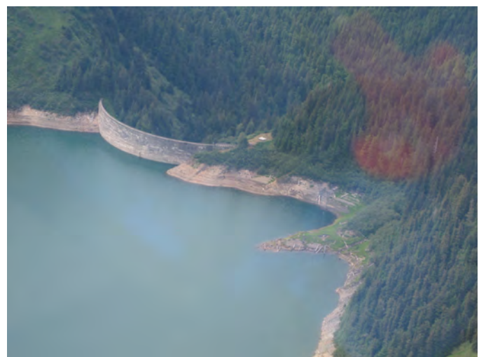
The Salmon Creek dam, built in Juneau in 1914, was the first variable radius arch dam in the world. The reservoir continues to provide drinking water and power for the city of Juneau. Photo by Nvvchar.
