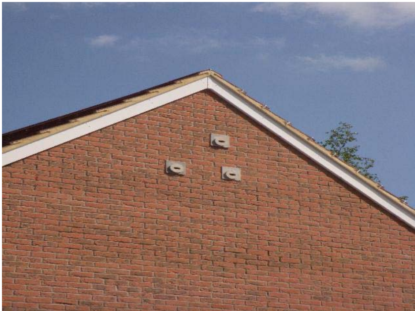
Plate 3. Internal Swift boxes with external cavity panels. (Photograph by Rob Mungovan) (See article on page 71)
