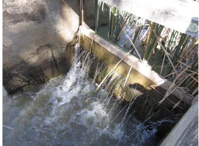
Camerons Creek regulator (Photo: C. Corr)
