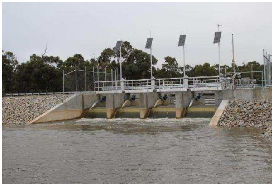
Hipwell Road Channel (Photo: A.Chatfield)
