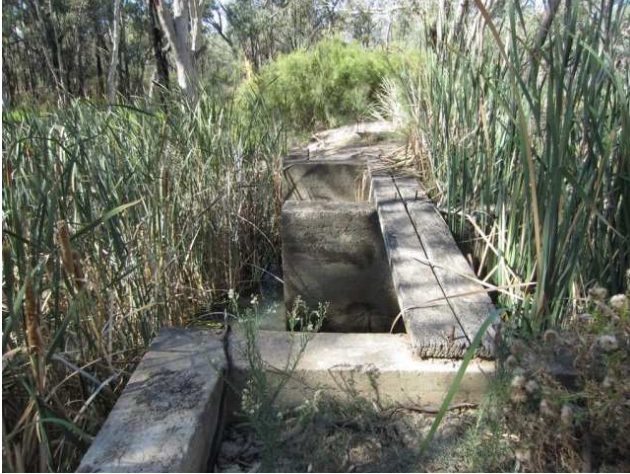
Camerons Creek regulator (Photo: C. Corr)
