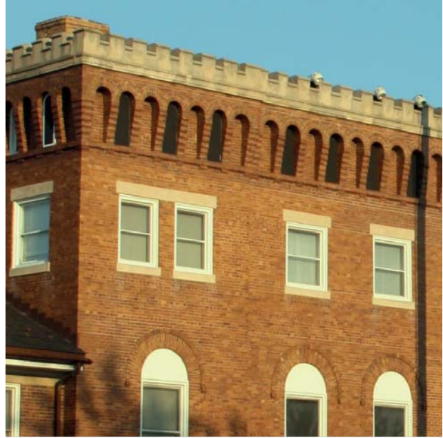
Future development at MBW should reflect and reinforce the existing architectural style and character of the historic campus.
