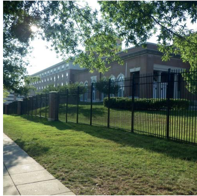
Large AT/FP standoff distances shown here at the MBW Annex (Bldg. 25) is a stark contrast to its urban context and the historic Main Post.
