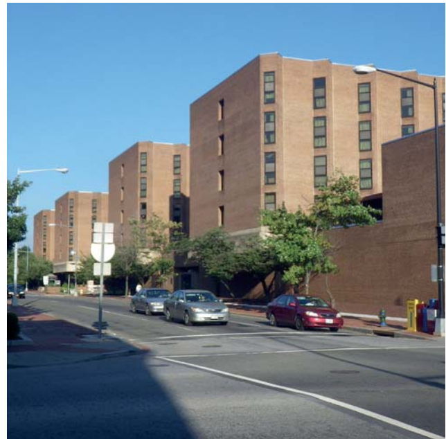
The proposed replacement BEQ will relocate function within Building 20 (above) and Building 9 at the Main Post.
