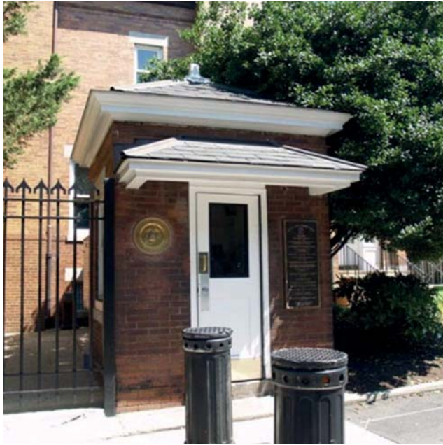
Building 10, vehicle and pedestrian sentry house at the Main Post.
