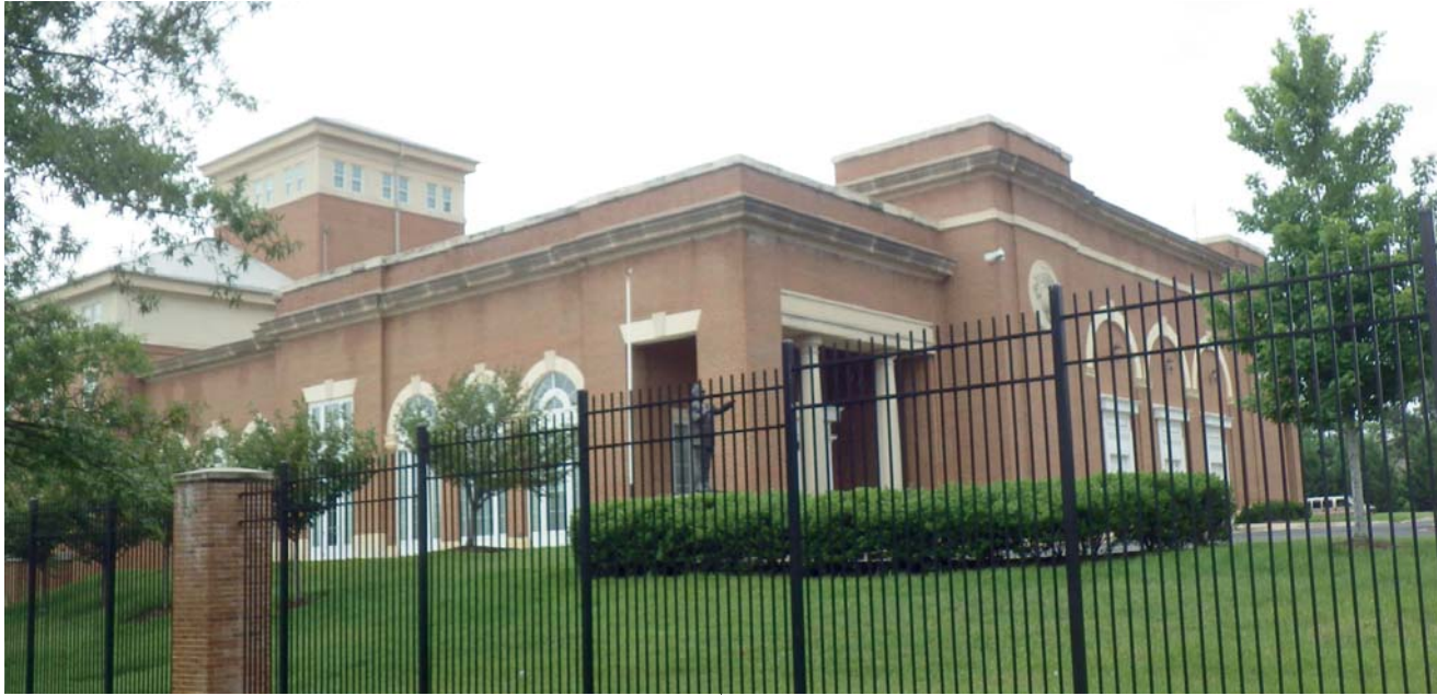
Flat roofs, such as Building 25, offer the greatest opportunity for incorporating solar panels at MBW with the least visual impact.
