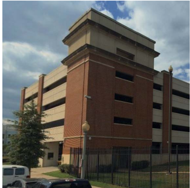
Building 26 at the MBW Annex illustrates the consistent use of materials, massing, and fenestration applicable for structured parking on the installation.
