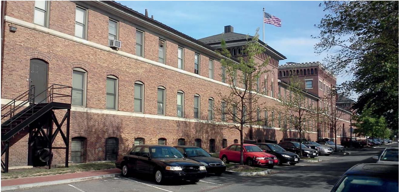
Non-compliant parking along 9th Street is within 17 feet of Building 8 and lacks a controlled perimeter.
