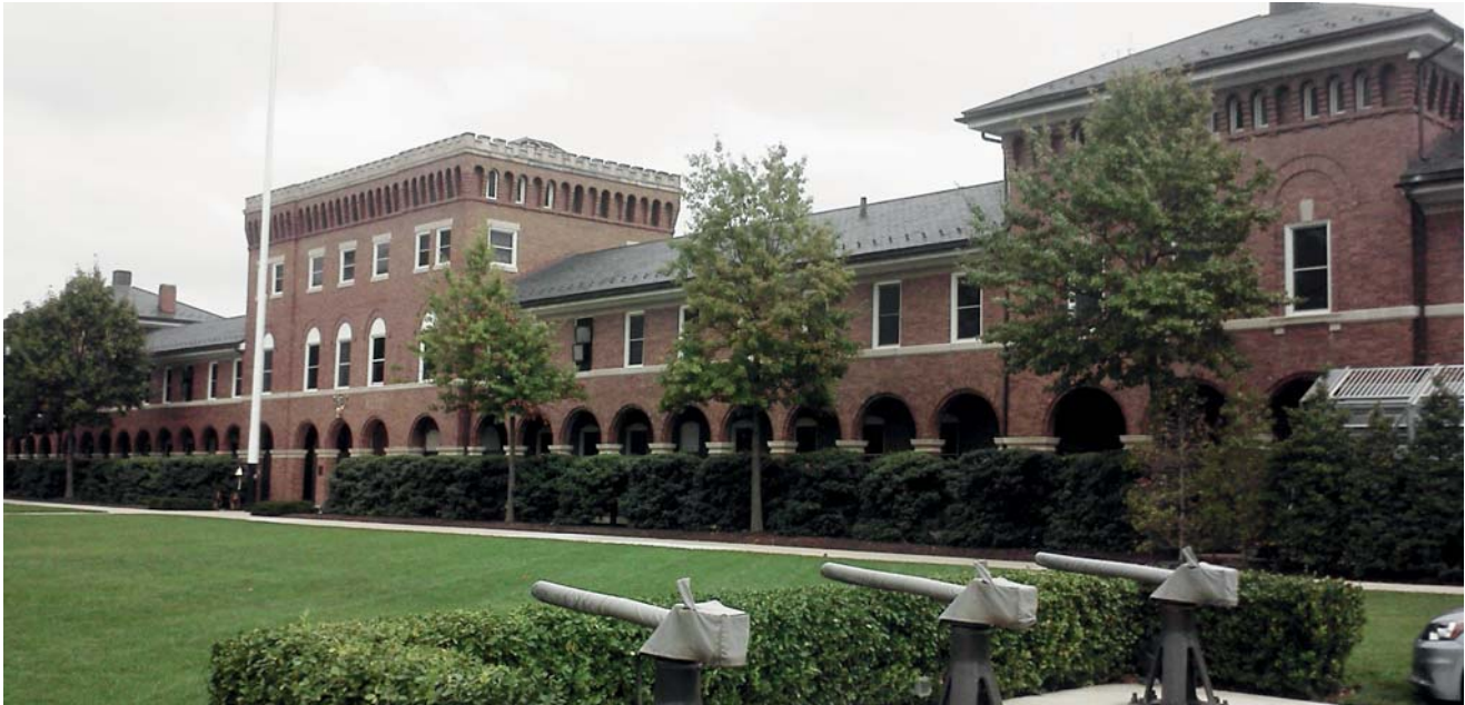
Building 8 at the Main Post exemplifies the historic use of fenestration at MBW, illustrating the range of scale, style, and placement that is consistent across the installation.
