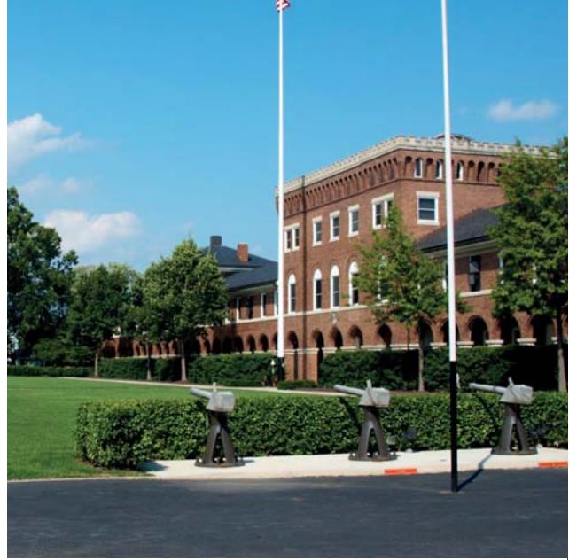
Historic Barracks Parade Ground at the Main Post functions as the ceremonial center for the installation along with serving as an effective pervious surface for SWM.
