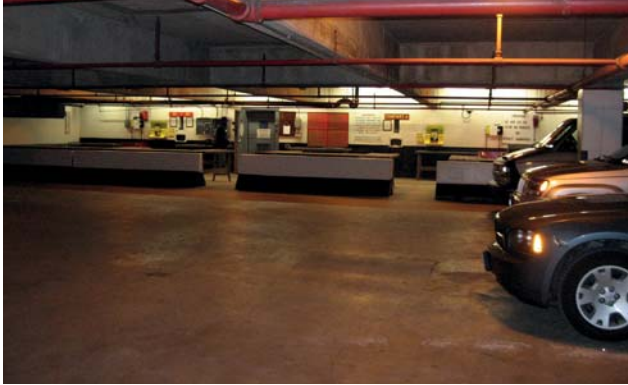
Building 20 houses over 200 below-grade parking spaces under the existing BEQ and support uses.
