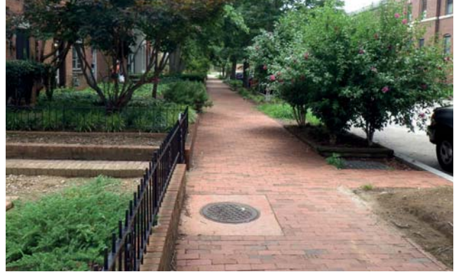
Sidewalk construction or restoration within designated historic districts must be constructed to be as consistent and compatible with the existing context as possible.
