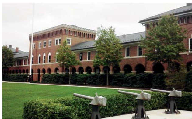
Housing close to 48,000 SF, the Command Post (Building 8) is MBW's largest administrative facility at MBW.
