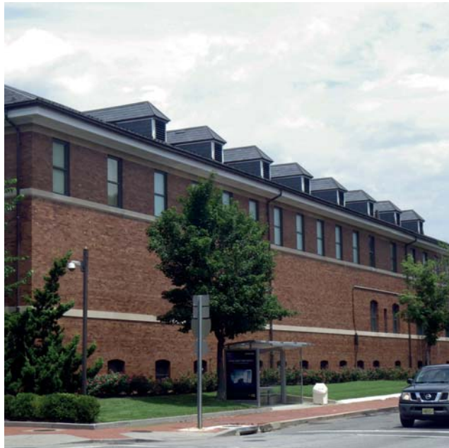
Multiple planning efforts are needed for Building 9 going forward including AT/FP compliance, space optimization, and potential of hazardous materials.
