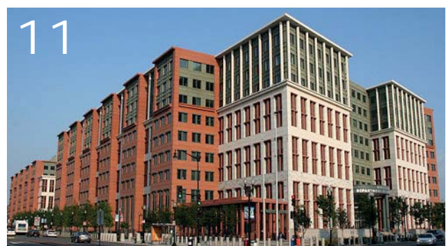
The 1.1-MSF USDOT headquarters building was completed in the spring of 2007 on a previous 11-acre portion of the Southeast Federal Center site.
