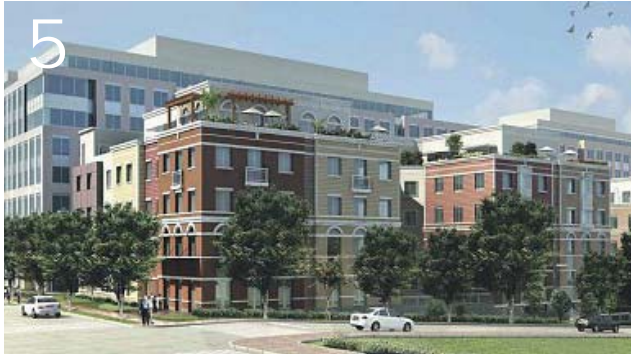
The Lofts at Capitol Quarter are under construction and projected to open in 2016 with 195 units at 7th and L Streets SE.
