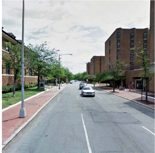
Building 20's barren streetscape is the focus of a near-term installation improvement project to introduce pedestrian scale design elements and signage.
