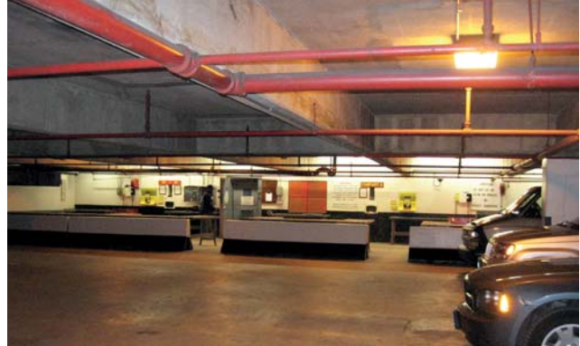
Building 20 parking garage.
