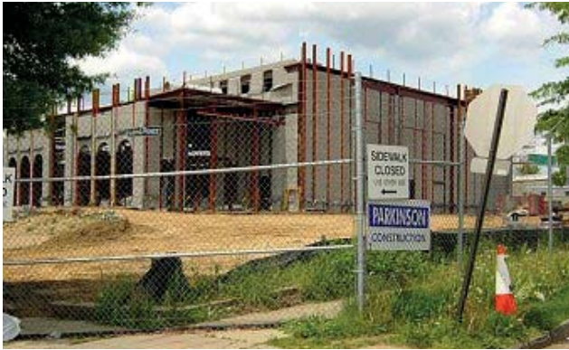
MBW Annex construction was completed in 2006.
