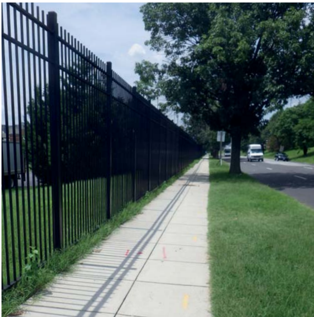
Annex development, while AT/FP compliant, lacks the visually consistent urban edge exemplified in the surrounding historic Capitol Hill community.
