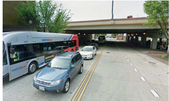
8th Street SE underpass (View facing south).
