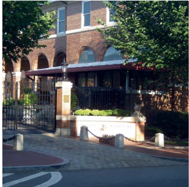
Driveway crossings should be at grade, of compatible material and design, and not obstruct public access.
