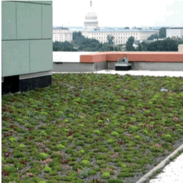
Low profile green roofs provide multiple benefits without visual impacts (shown: DDOT Headquarters).
