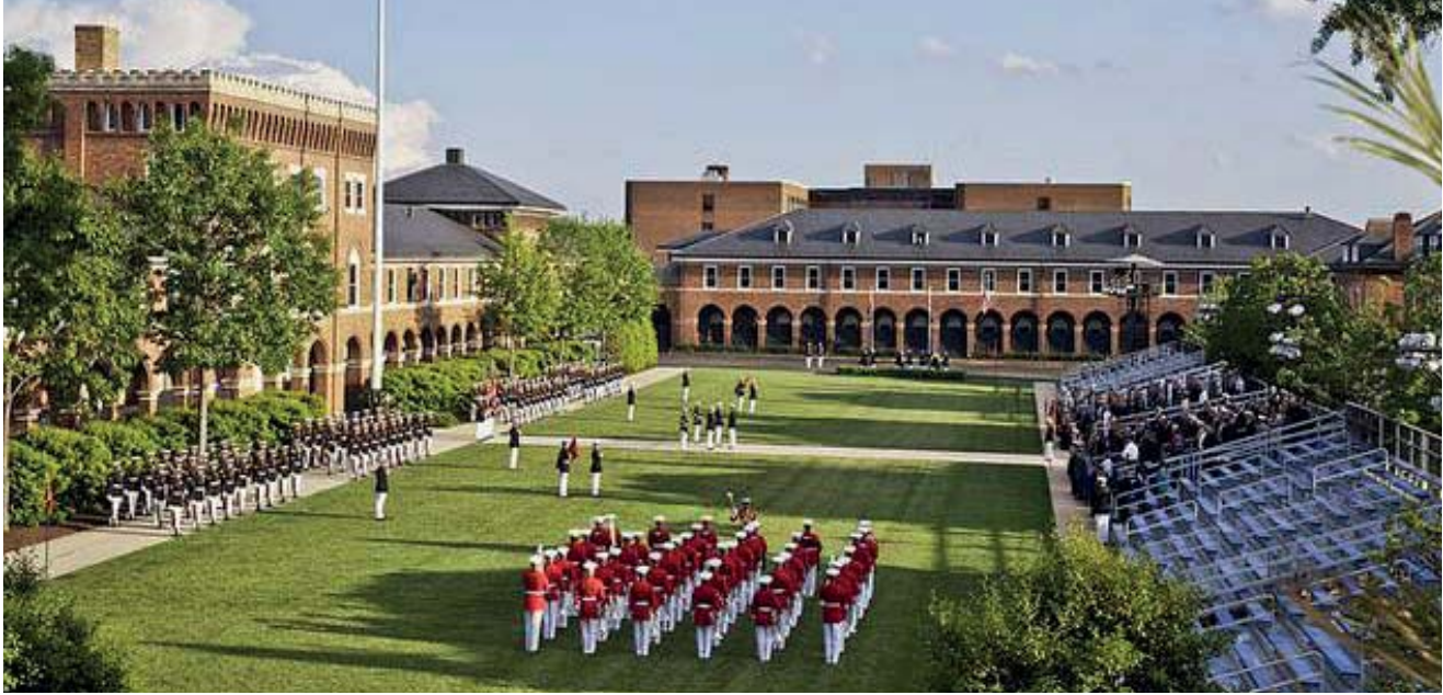
View south of the ceremonial parade ground at MBW Main Post.
