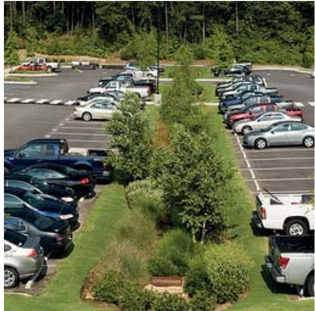
Example of a bioswale incorporated into a parking area.
