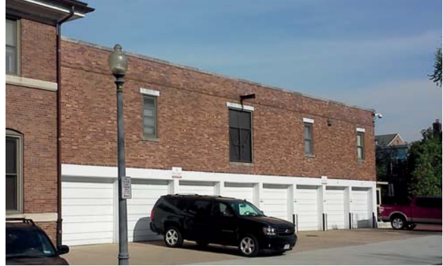
The ground floor of Building 7 houses eight POV parking spaces for on-site SOQ and GOQ residents.
