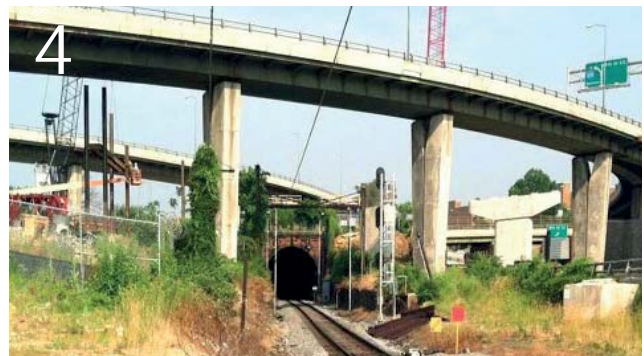
CSX Virginia Avenue Tunnel Expansion will increase capacity between 2nd and 11th Streets SE, adjacent to MBW Annex (Virginia Avenue).
