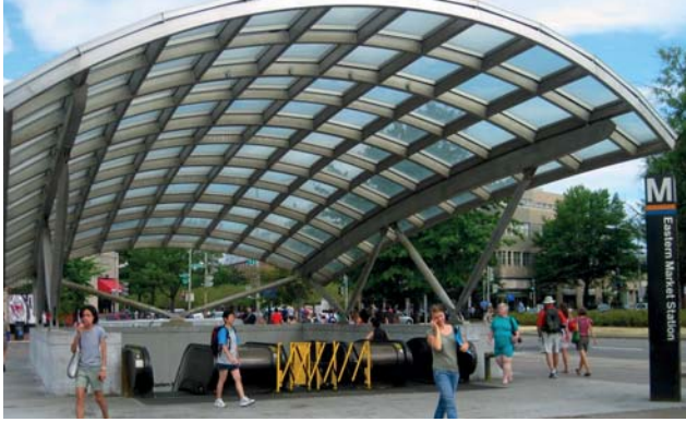
Eastern Market Metro Station is approximately a 10-minute walk north of MBW along 8th Street.
