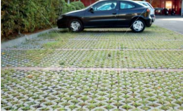
Pervious pavement comes in many forms and applications designed to reduce SWR and increase infiltration rates while providing stability and low maintenance.
