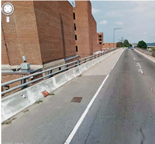
Building 20 is located just 13 feet from the adjacent Southeast Freeway on-ramp.
