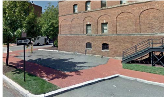
Special pavement at Building 8 lacks consistency with surrounding uses.
