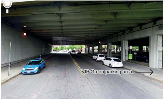
7th Street SE underpass (View facing north).
