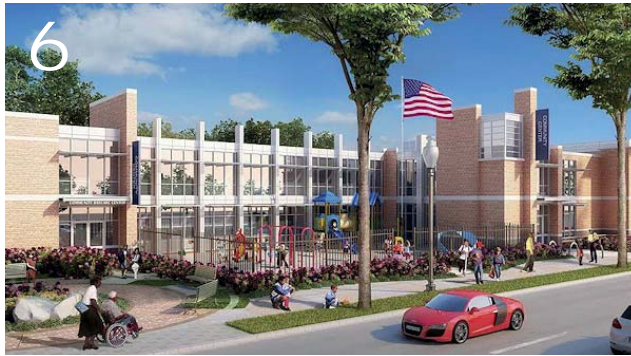
Capitol Quarter Community Building is under construction west of the Annex parking garage.
