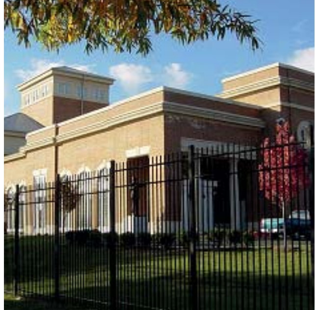
Housing and Community Support (Facility Category 100) encompasses the largest facility footprint at MBW.
