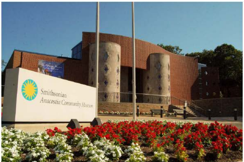
VISITORS' ENTRANCE: VIEW SOUTHEAST FROM MAIN ENTRANCE
