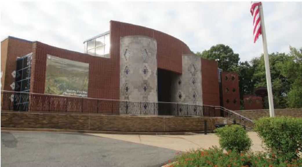
EXISTING BUILDING FACADE & LANDSCAPE MATERIALS
