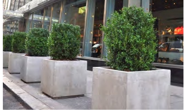
Reinforced planters can provide aesthetic solution to site security.
