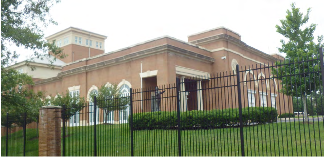
Flat roofs, such as Building 25, offer the greatest opportunity for incorporating solar panels at MBW with the least visual impact.
