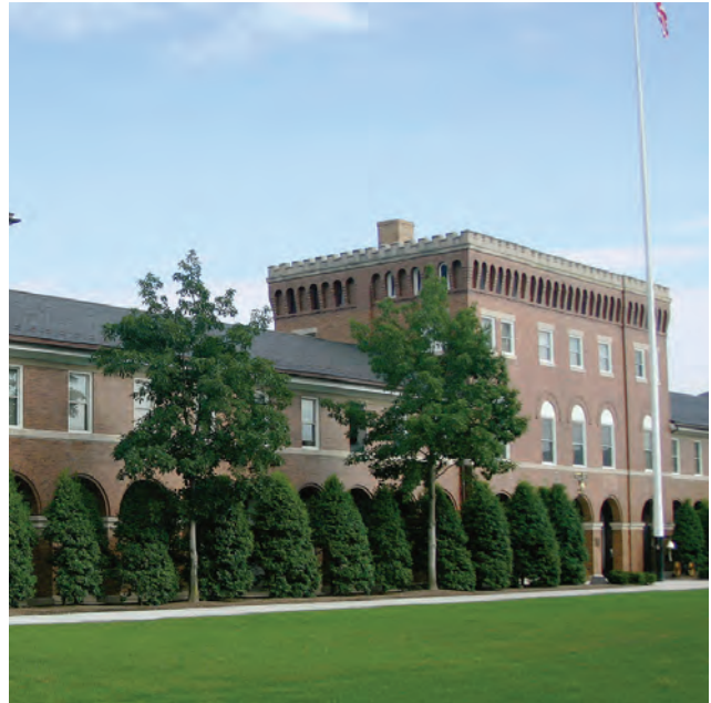
The Main Post serves primarily as the administrative hub, anchored by the Installation Command Post (Building 8).
