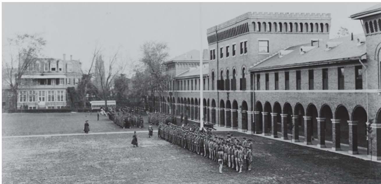
Barracks (Building 8) at the Main Post, circa 1917.
