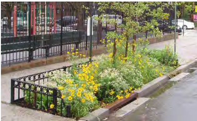
Vegetated strips slow runoff and increase infiltration as well as enhance the aesthetics of the urban streetscape.
