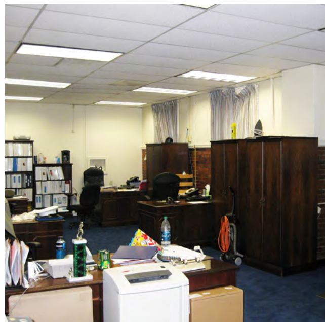
Building 8 is long overdue for interior renovations to address multiple deficiencies in major building systems and space utilization.
