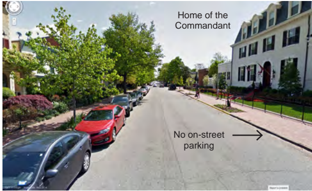
G Street SE (Residential character, view facing east).
