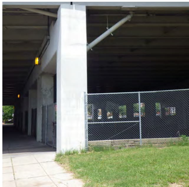
IAP improvements include consistent treatment of fencing, pavement, signage, landscape, and other design elements at the VIP Green that enhance campus continuity.
