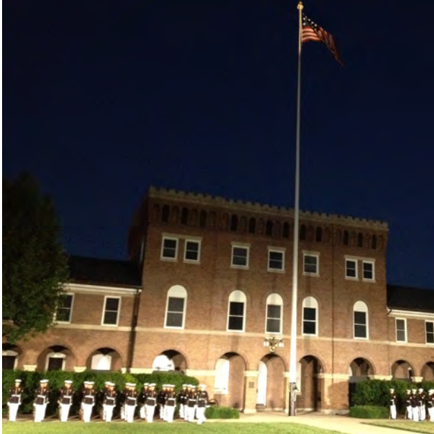
The greatest opportunity for maximizing the existing space at MBW includes the repair and renovation of historic facilities at the Main Post (Building 8 shown above).
