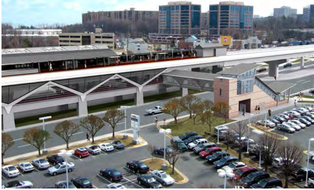
Five Silver Line Metrorail stations opened to the public in July 2014 connecting Tysons Corner and Reston, Virginia to Downtown DC and MBW via the Eastern Market Station.
