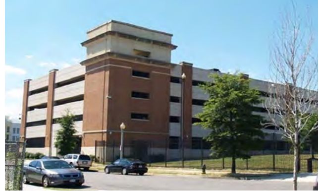
Structured parking (CCN 85310) is the largest building use at MBW, comprising nearly one third of the total facility footprint.
