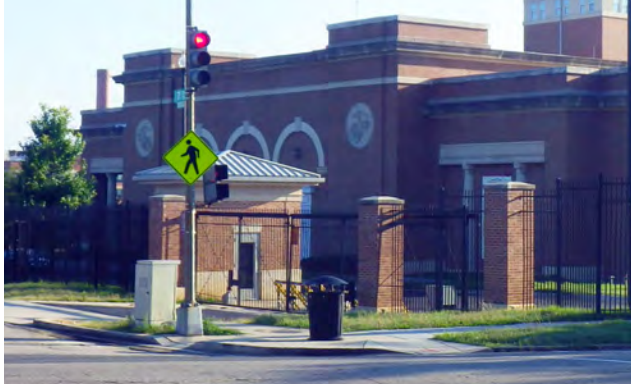
Main pedestrian entrance at the Annex lacks character and branding.
