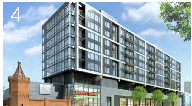
Recently constructed Harris Teeter site (Parcel D) provides 50,000 SF of ground level retail along M Street.
