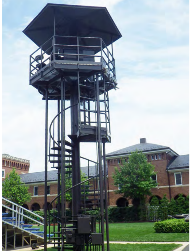
Building 23 south tower, one of two observation structures overlooking the parade ground at the Main Post.
