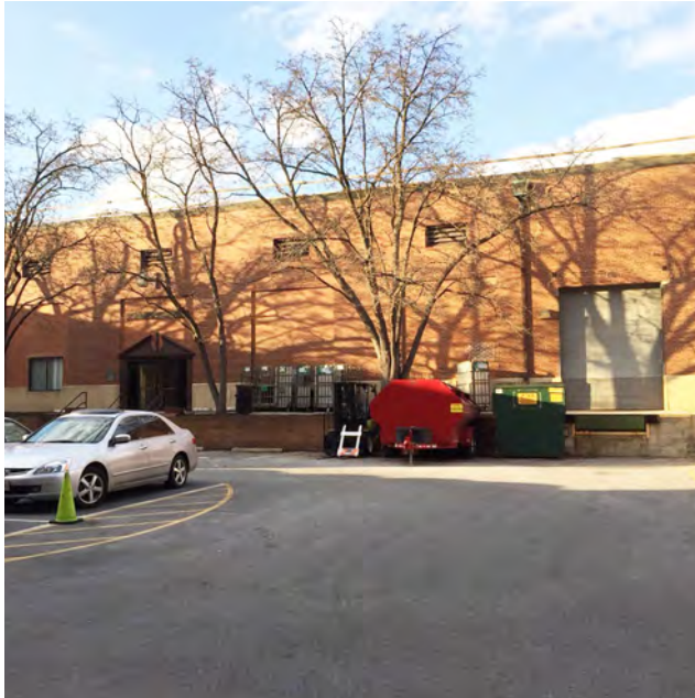
View facing north from parking lot serving Building 169.
