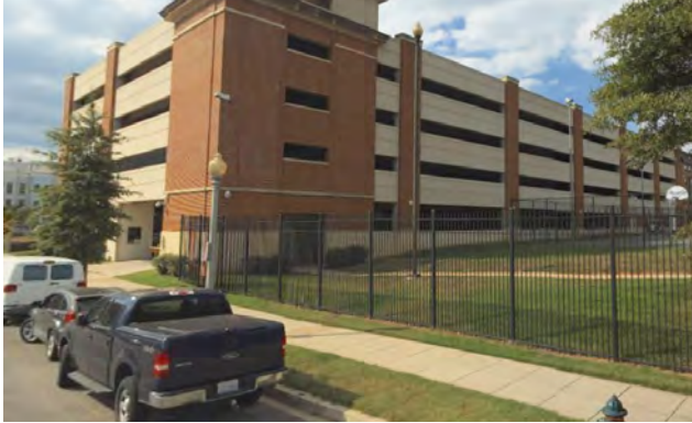
View of Site E facing northwest towards the existing parking garage (Building 26).
