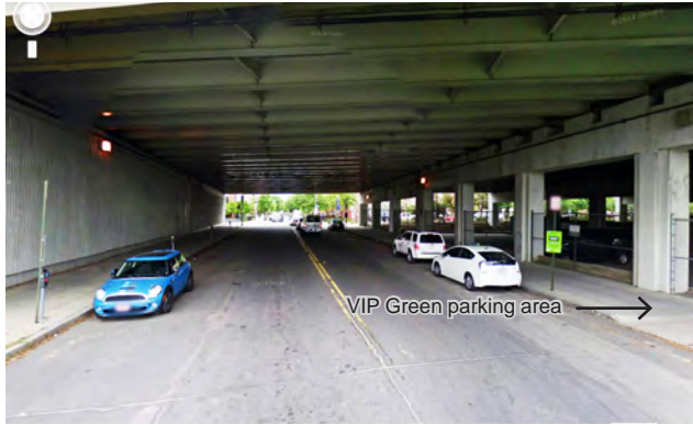
7th Street SE underpass (View facing north).
