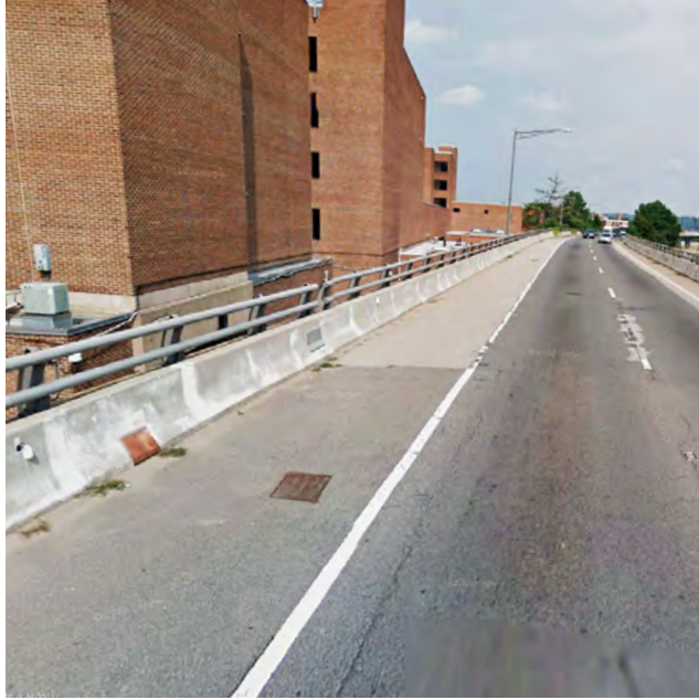
The south façade of Building 20 lies within 13 feet of the Southeast Freeway.
