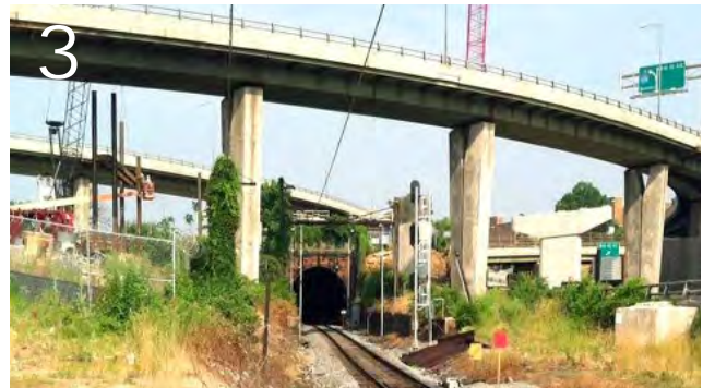
CSX Virginia Avenue Tunnel Expansion will increase capacity between 2nd and 11th Streets SE, adjacent to MBW Annex (Virginia Avenue).
