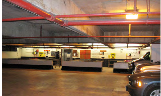
Building 20 parking garage.
