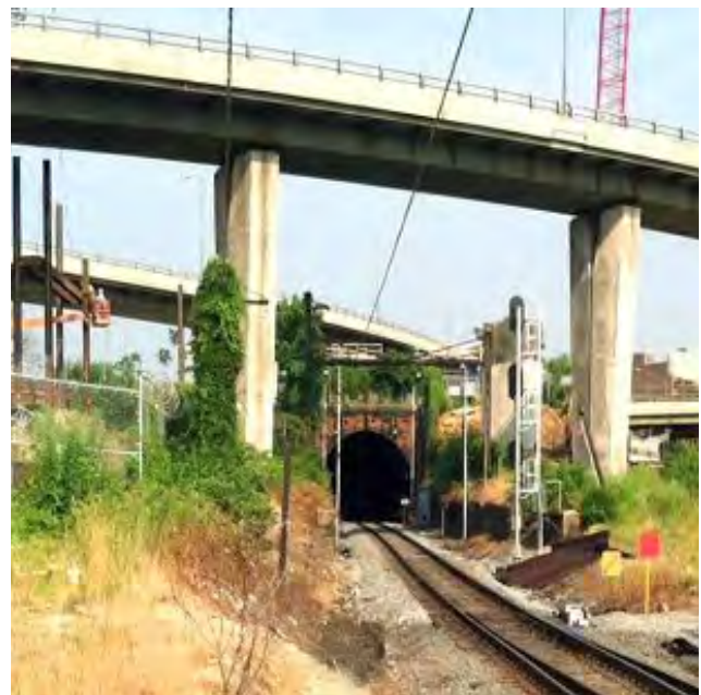
Existing Virginia Avenue tunnel (11th Street entrance).
