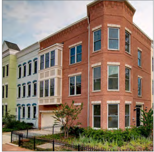
Capper Carrollsburg housing located west of MBW Annex.
