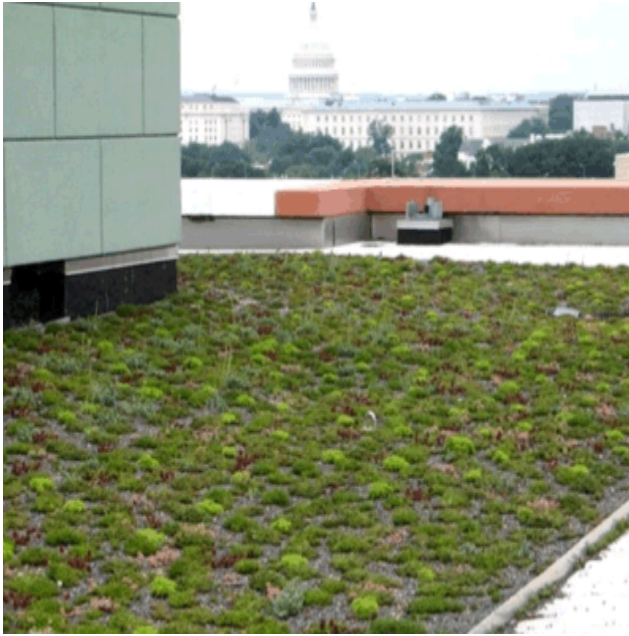
Low profile green roofs provide multiple benefits without visual impacts (shown: DDOT Headquarters).
