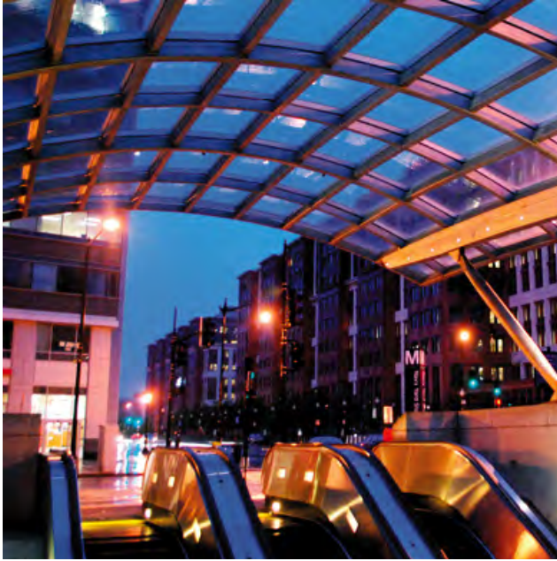
Navy Yard Metrorail Station exiting onto M Street SE is roughly an 8- to 10-minute walk from MBW.
