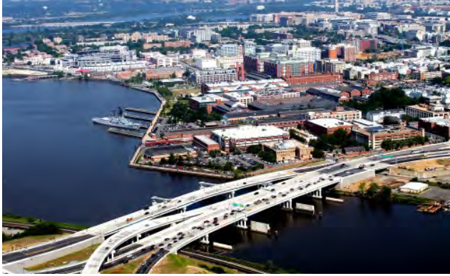
11th Street Bridge crossing the Anacostia River near WNY.
