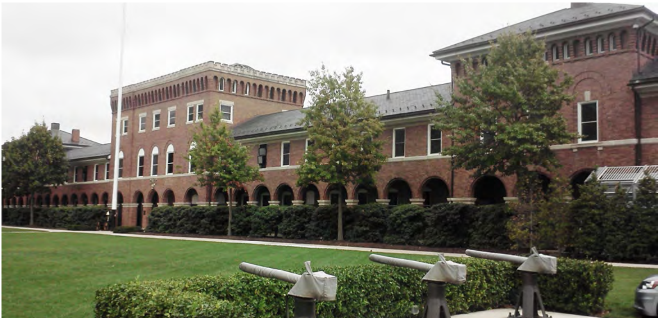
Building 8 at the Main Post exemplifies the historic use of fenestration at MBW, illustrating the range of scale, style, and placement that is consistent across the installation.
