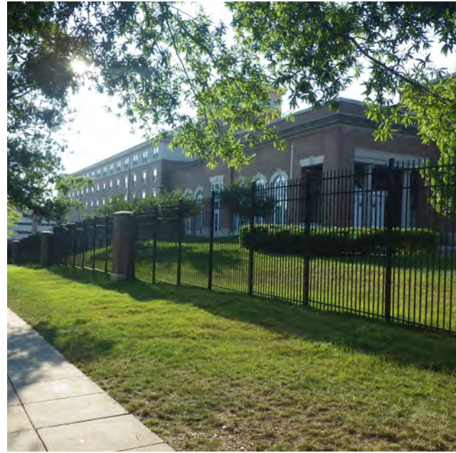
Large AT/FP standoff distances shown here at the MBW Annex (Bldg. 25) is a stark contrast to its urban context and the historic Main Post.
