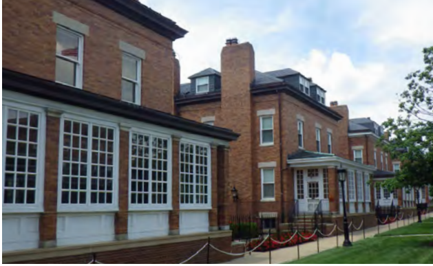
Senior Officers Quarters (SOQ) 1 through 5 provide repeating symmetry and a residential scale to the western boundary of the Main Post.
