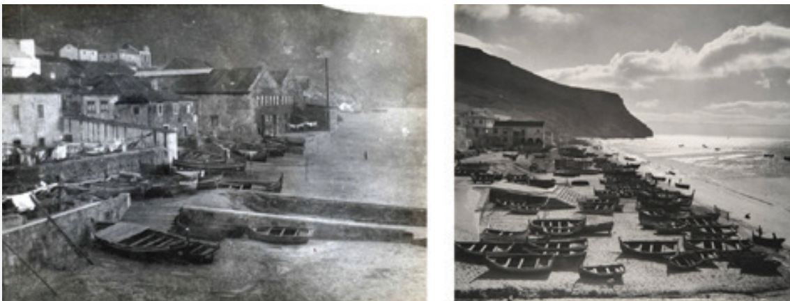
Figure 3: Protection walls, piers and ramps in the Sesimbra waterfront, early XXth century. (unknown author; Artur Pastor)
