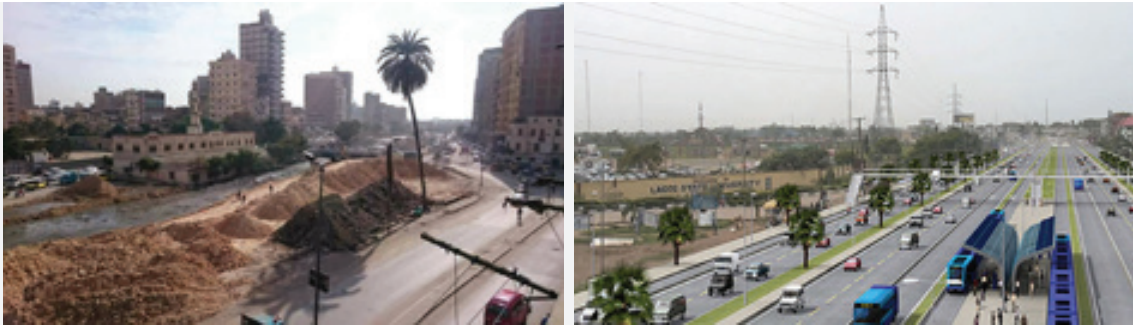
Figure 1: left. The Mahmoudia Canal during the filling up process now, right. Abuja new highway, Nigeria. Proposed as a similar concept of “New Mahmoudia Line” Source: left: by researchers, right:( http://moovafrika.com/news/nigerias-average-fare-up-23-99-month-on-month-inter-city-transport-fares-show-abuja-cross-river-jigawa-in-the-lead-nbs-report/ )
