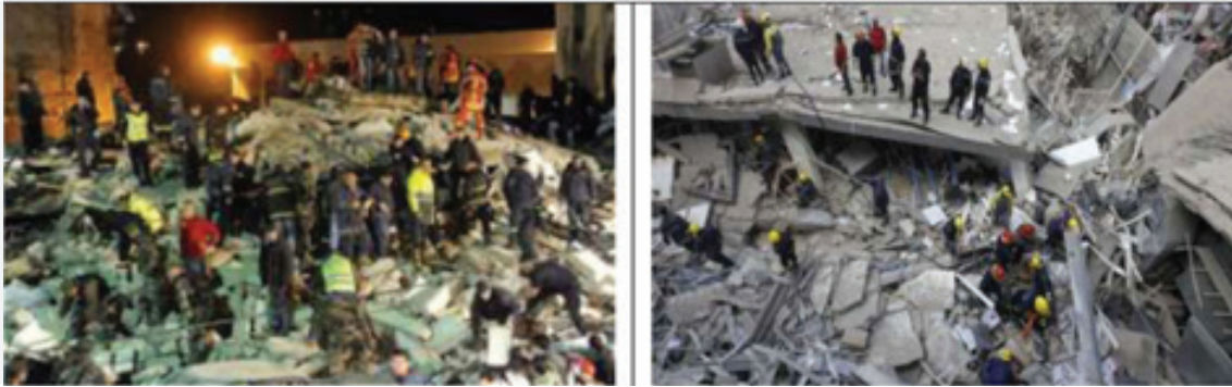
Figure 1: a-Building collapse and debris scattering b-Truncated pyramid shape of debris
