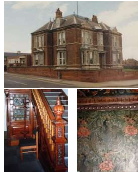
The Knoll (1898), Alexandra Road, Grade II, described by Pevsner as a 'prosperous house'.
