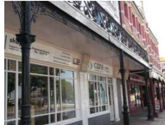
Image of the cast iron balcony over 46 and 47 Alexandra Road.
