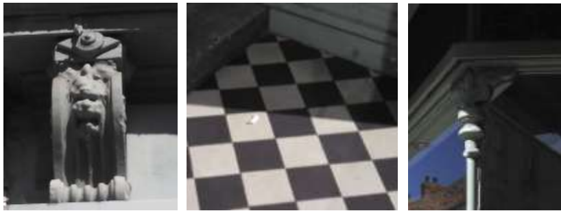
Images of 24 Seaview Street. (Left) Corbel in classical leaf and grape design. (Central) Tiled entrance. (Right) Column window frame.
